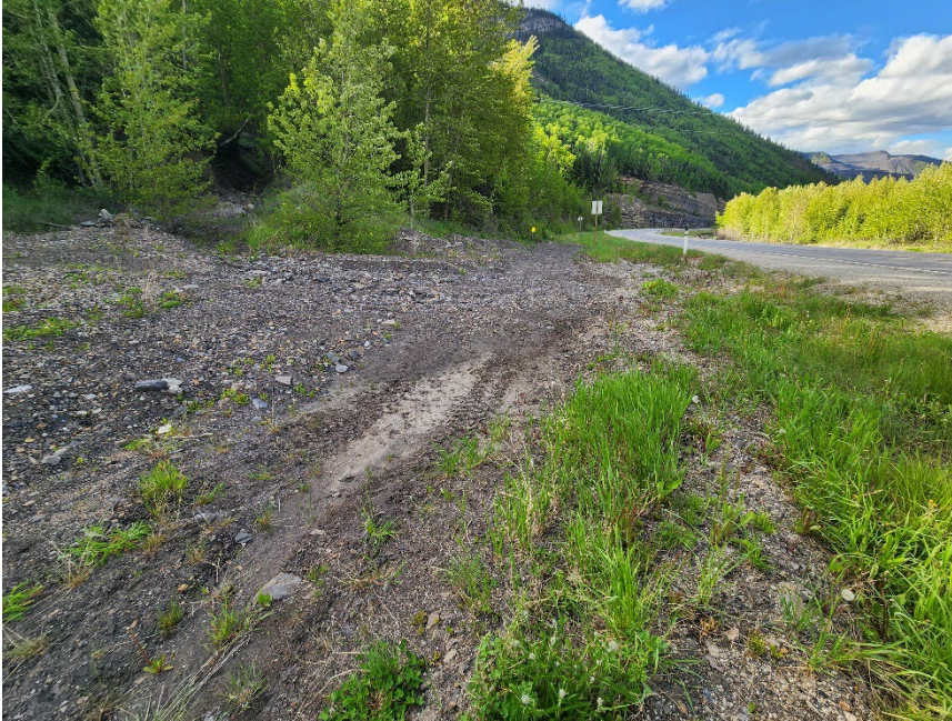
Photo 2 Debris flow at km 8.1 on west side of Hwy 40:36. Note erosion gully is approximately 4 m high. Photo taken June 10, 2024, facing northwest.
