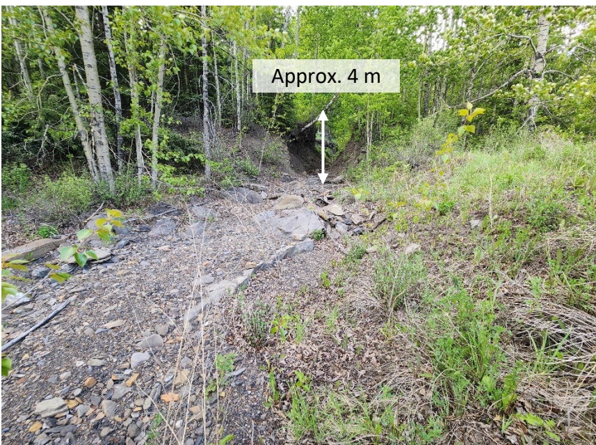
Photo 2 Debris flow at km 8.1 on west side of Hwy 40:36. Note erosion gully is approximately 4 m high. Photo taken June 10, 2024, facing northwest.
