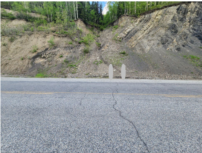
Photo 8 Debris flow at km 12.1 on west side of Hwy 40:36. Note erosion gully near middle of debris flow fan. Photo taken June 10, 2024, facing northwest.
