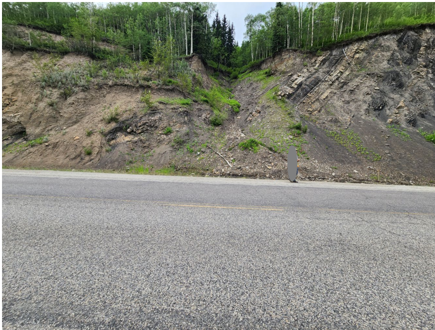
Photo 6 Debris flow at km 12.1 on west side of Hwy 40:36 at WP300. Note erosion gully down debris fan and water at toe of debris flow in highway ditch. Photo taken June 12, 2023, facing west.
