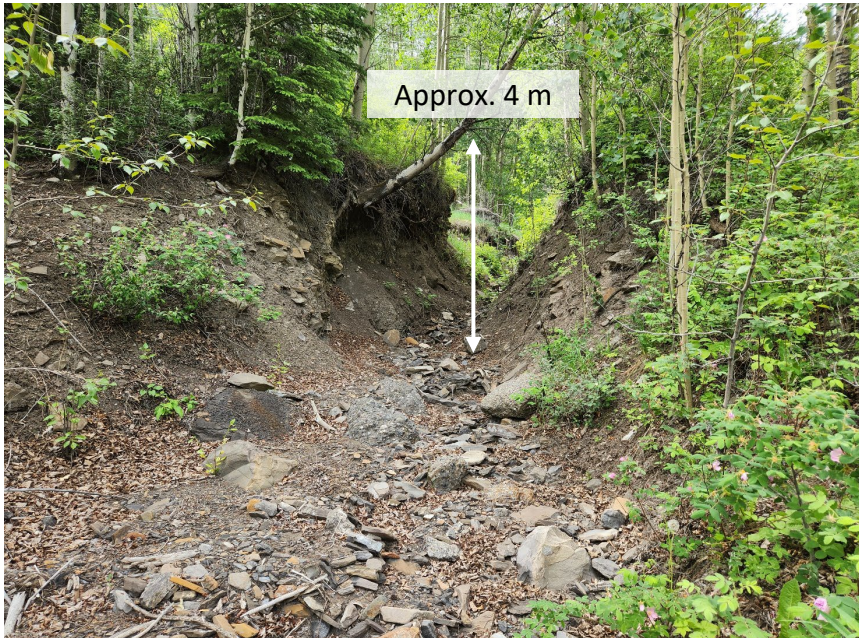
Photo 2 Debris flow at km 8.1 on west side of Hwy 40:36 at WP296. Note debris fan (mostly sand and gravel with some cobbles) in highway ditch. Photo taken June 12, 2023, facing northwest.
