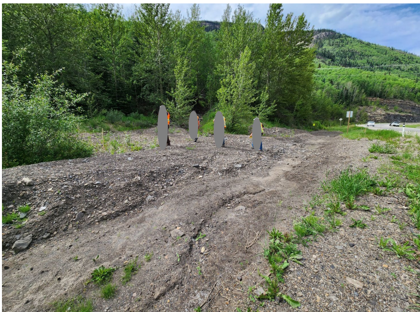
Photo 2 Debris flow at km 8.1 on west side of Hwy 40:36 at WP296. Note debris fan (mostly sand and gravel with some cobbles) in highway ditch. Photo taken June 12, 2023, facing northwest.
