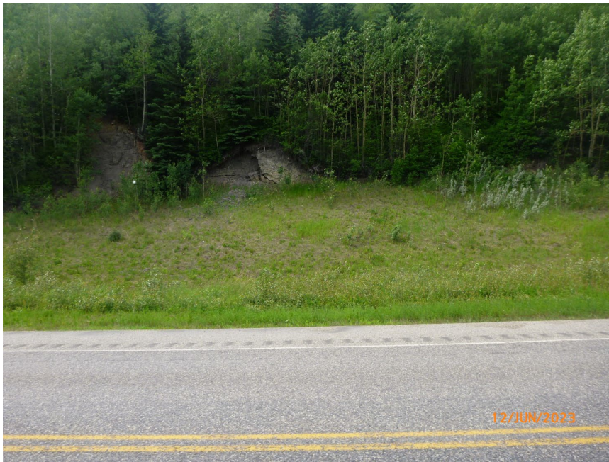
Photo 6 Debris flow at km 12.1 on west side of Hwy 40:36 at WP300. Note erosion gully down debris fan and water at toe of debris flow in highway ditch. Photo taken June 12, 2023, facing west.
