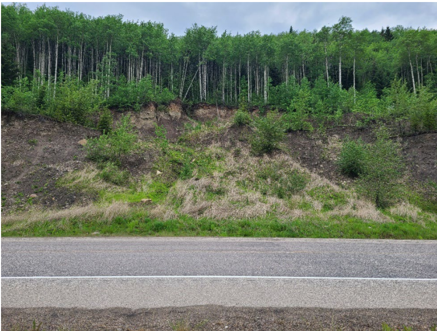
Photo 8 Debris flow at km 11.2 along backslope on west side of Hwy 40:36 at WP188. Photo taken June 14, 2022, facing west.
