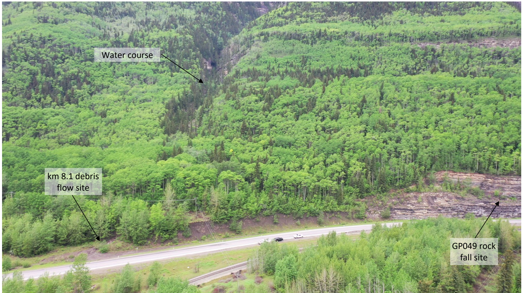
Photo 2 Debris flow at km 8.1 along backslope on west side of Hwy 40:36. Note water course above debris flow location. Photo taken June 14, 2022, facing west.
