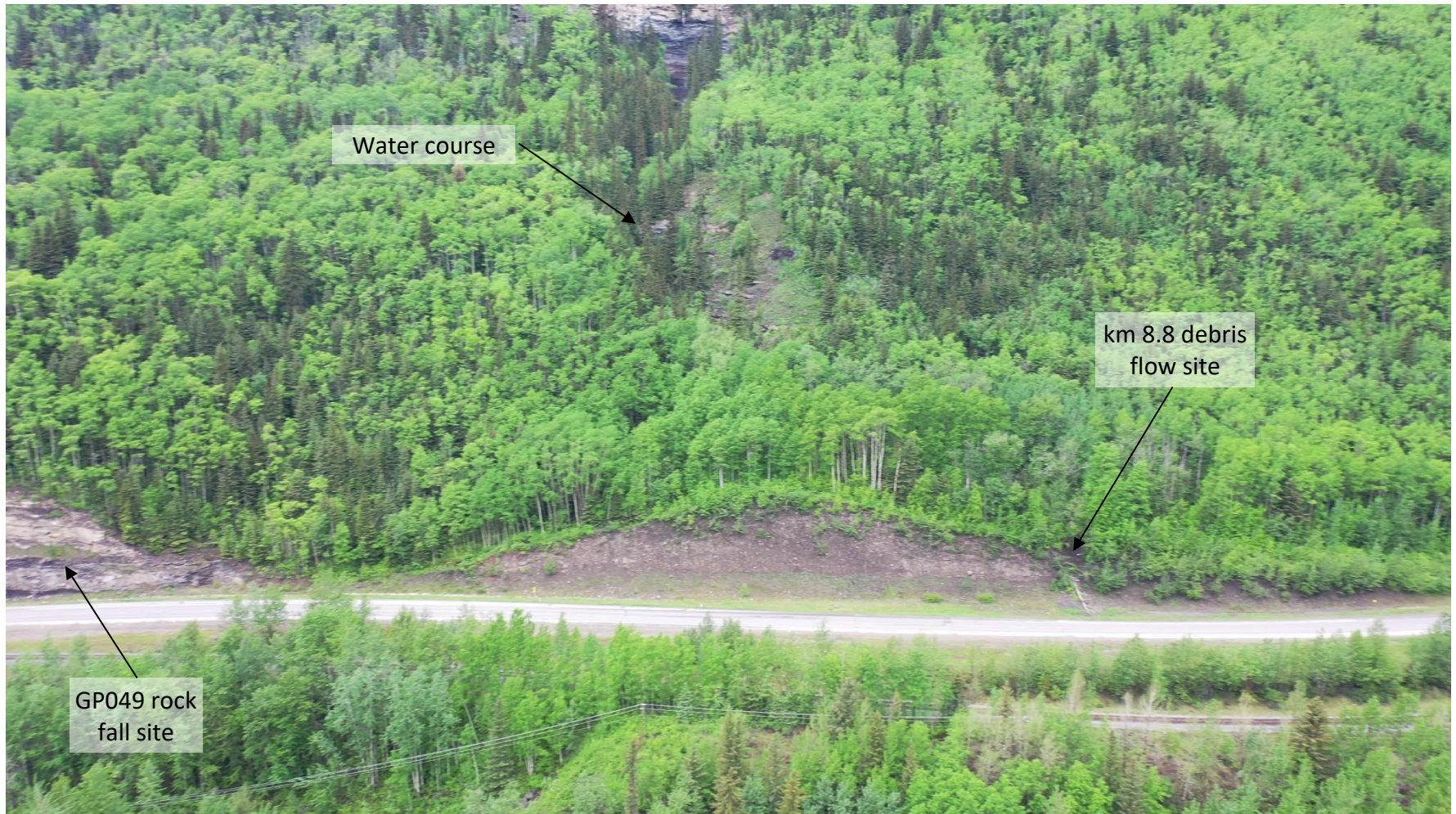
Photo 3 Debris flow at km 8.8 along backslope on west side of Hwy 40:36. Note water course above debris flow location. Photo taken June 14, 2022, facing west.
