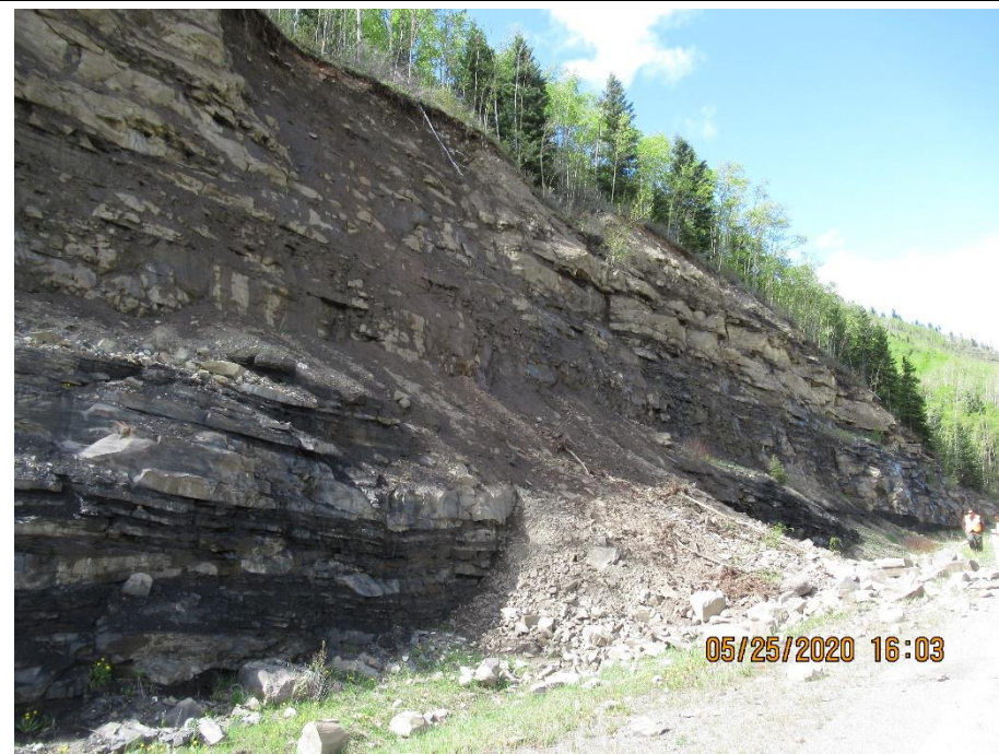
Photo 2. Hwy 40:36 km 8.5 Looking northwest up at the backslope face just to the north of Photo 1. Note that there appear to be a couple of older, smaller debris deposits that have accumulated in the ditch.
