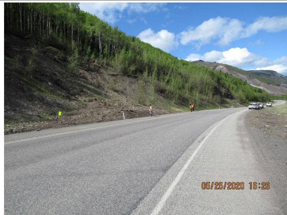
Photo 16. Hwy 40:36 km 11.2 Looking northwest from NBL shoulder across Hwy 40:36 towards slide mass.
