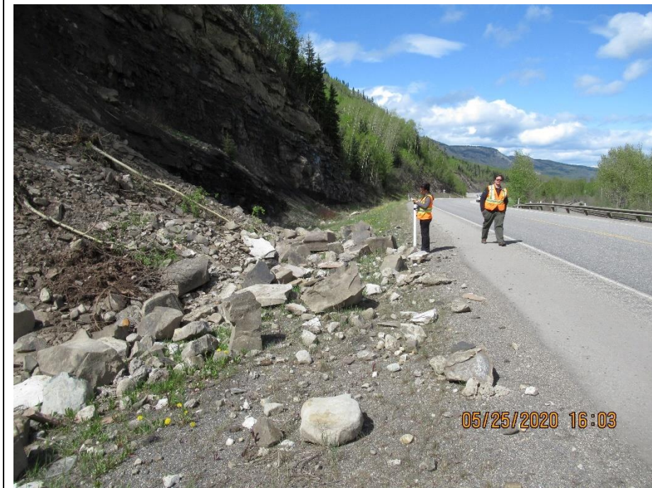
Photo 4. Hwy 40:36 km 8.5 Looking northeast from the shoulder of the EBL of Hwy 40:36 at the fallen rocks on the highway shoulder.
