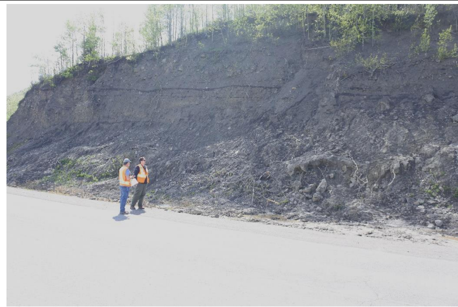
Photo 14. Hwy 40:36 km 11.2 Looking southwest across Hwy 40:36 at debris which has fallen down.
