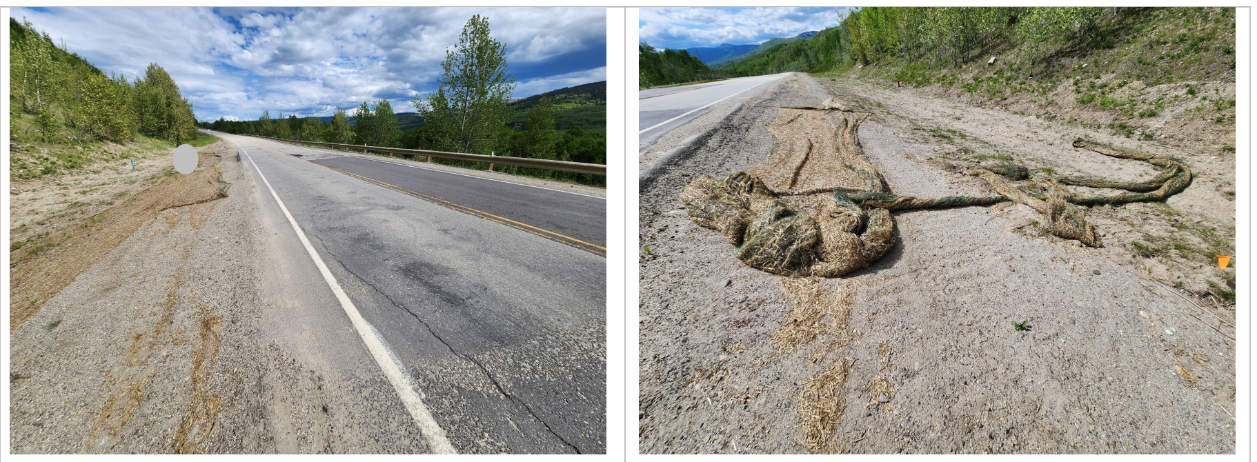
Photo 3 Ditch on north side of Hwy 40:36 near west end of GP007 site. Ditch was regarded in fall 2023. Note rolled erosion control product unsecured from ground. Photos taken June 10, 2024, facing east and west, respectively.
