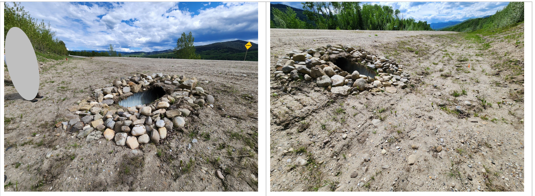
Photo 3 Ditch on north side of Hwy 40:36 near west end of GP007 site. Ditch was regarded in fall 2023. Note rolled erosion control product unsecured from ground. Photos taken June 10, 2024, facing east and west, respectively.
