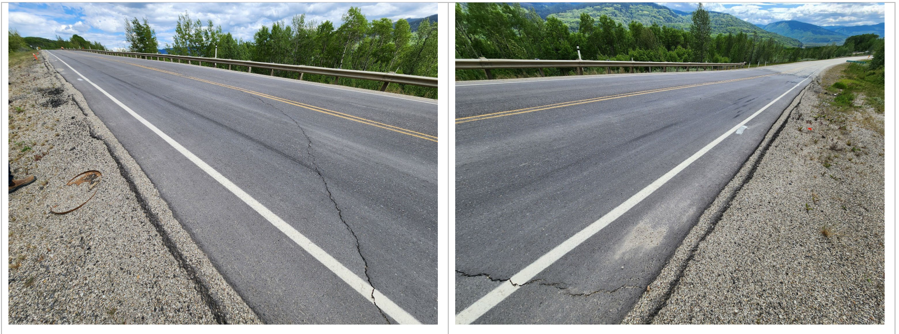
Photo 7 Cracking and settlement across Hwy 40:36 near middle of recent pavement patch at east end of GP007 site. Photos taken June 10, 2024, facing west and northeast, respectively.
