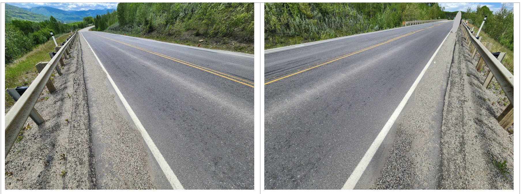
Photo 7 Cracking and settlement across Hwy 40:36 near middle of recent pavement patch at east end of GP007 site. Photos taken June 10, 2024, facing west and northeast, respectively.
