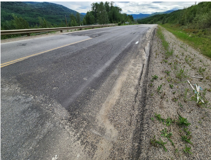
Photo 4 Cracking and settlement of recent pavement patch in both lanes of Hwy 40:36 near western site limit. Photo taken June 12, 2023, facing west.
