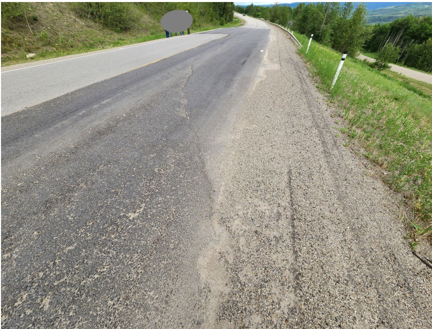
Photo 4 Cracking and settlement of recent pavement patch in both lanes of Hwy 40:36 near western site limit. Photo taken June 12, 2023, facing west.
