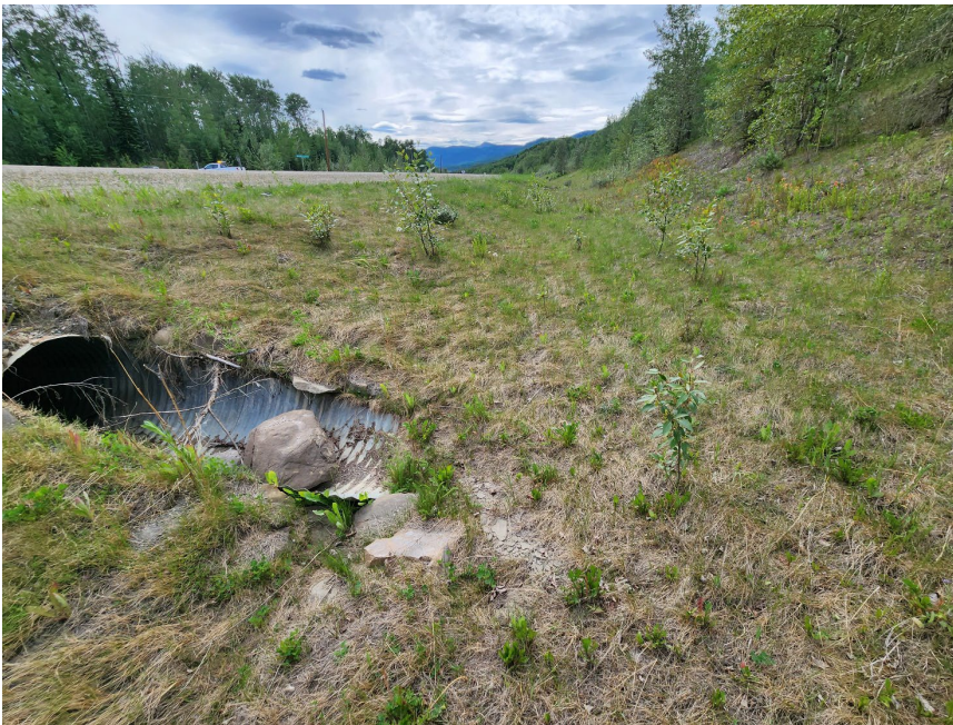
Photo 6 North ditch of Hwy 40:36 at western site limit near Wanyandie Road intersection. Note boulder-sized rock particle (approximate diameter 0.3 m) in culvert inlet. Photo taken June 12, 2023, facing west.
