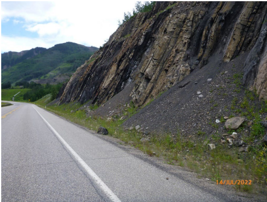
Photo GP053-I – 4 Different (second) structure of bedrock with different orientation of bedding planes. Note non-planar distortion of bedding planes in a gentle fold. The near vertical bedding plane bedrock structure shown in Photos GP053-2 is located at the lower lefthand corner of this photo. Photo taken July 14, 2022, facing northwest.
