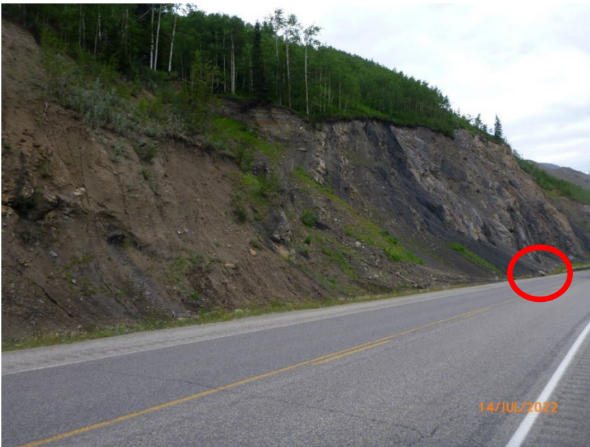
Photo GP036 – 2 Soil-infilled possible fault structure between rock slopes. South end of north part of site shown in this photo. Largest rock fall in July 2022 rainfall and rockfall event is shown by red circle. Photo taken July 14, 2022, facing northwest.
