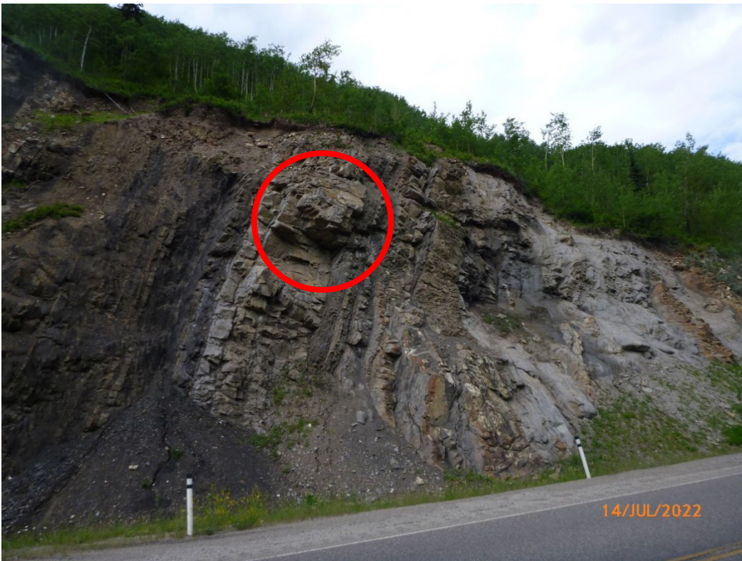
Photo GP036 – 14 Rock slope at north limit of rock cut slope. Red circle indicates overhang in upper third point of slope (shown in Photo -15). Photo taken July 14, 2022, facing northwest.
