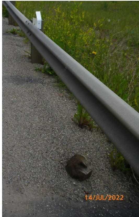
Photo GP053-I – 5 Rockfall particles under guardrail on opposite side of the highway from rock slope. Photos taken July 14, 2022, facing southwest and northeast respectively.
