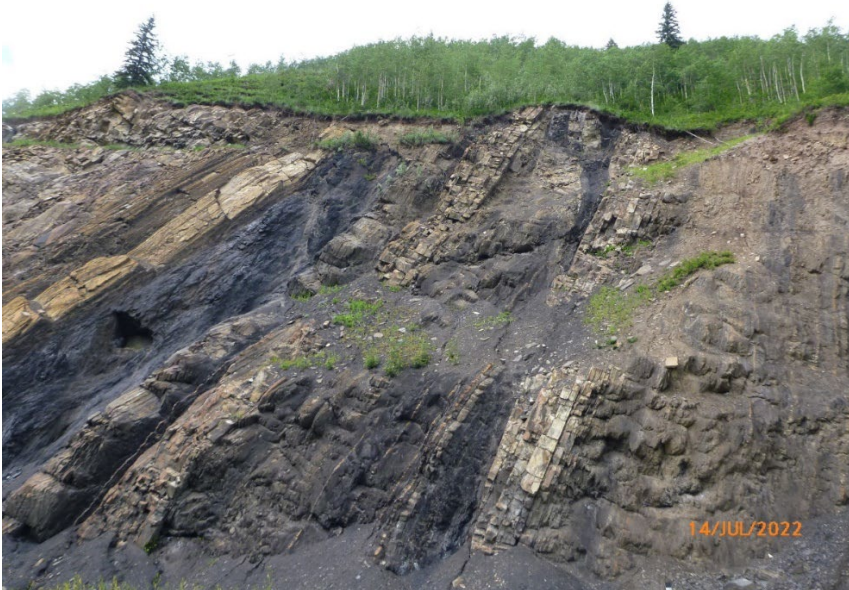
Photo GP036 – 14 Rock slope at north limit of rock cut slope. Red circle indicates overhang in upper third point of slope (shown in Photo -15). Photo taken July 14, 2022, facing northwest.
