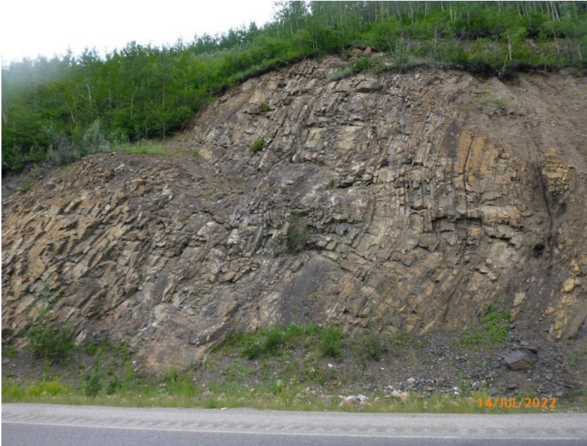
Photo GP036 – 2 Soil-infilled possible fault structure between rock slopes. South end of north part of site shown in this photo. Largest rock fall in July 2022 rainfall and rockfall event is shown by red circle. Photo taken July 14, 2022, facing northwest.
