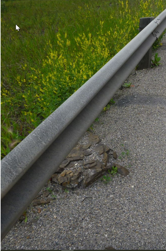
Photo GP053-I – 5 Rockfall particles under guardrail on opposite side of the highway from rock slope. Photos taken July 14, 2022, facing southwest and northeast respectively.
