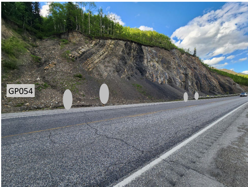
Photo 2 Rock slope along west side of Hwy 40:36. Note GP054 km 12.1 debris flow site on left and talus material mainly from coal seams in ditch. Photo taken June 10, 2024, facing northeast.
