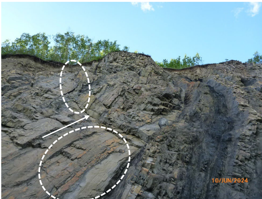
Photo 4 Potential rock block on upper slope shown in previous photo. Note dilated or open joints below rock block (indicated with white arrow), joints or shear planes to left and below rock block (circled in white), and rock and coal to right of rock block which is eroding. Photo taken June 10, 2024, facing northwest.
