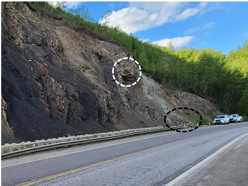
Photo 8 Rock slope along west side of Hwy 40:36 near north end of site. Note hanging rock block (circled in white) and rockfall that occurred between 2023 and 2024 inspections (circled in black, see next photo). Photo taken June 10, 2024, facing north.
