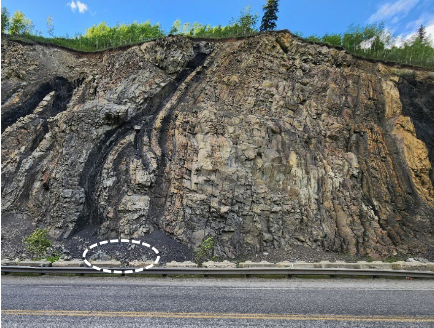
Photo 6 Rockfall particles in ditch on west side of Hwy 40:36. Note two larger particles circled in white fell between 2023 and 2024 inspections. Photo taken June 10, 2024, facing northeast.
