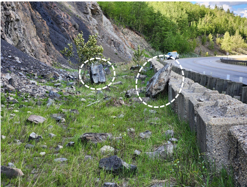
Photo 6 Rockfall particles in ditch on west side of Hwy 40:36. Note two larger particles circled in white fell between 2023 and 2024 inspections. Photo taken June 10, 2024, facing northeast.
