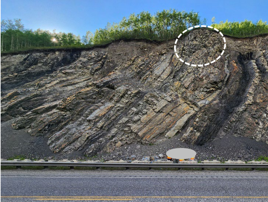
Photo 4 Potential rock block on upper slope shown in previous photo. Note dilated or open joints below rock block (indicated with white arrow), joints or shear planes to left and below rock block (circled in white), and rock and coal to right of rock block which is eroding. Photo taken June 10, 2024, facing northwest.
