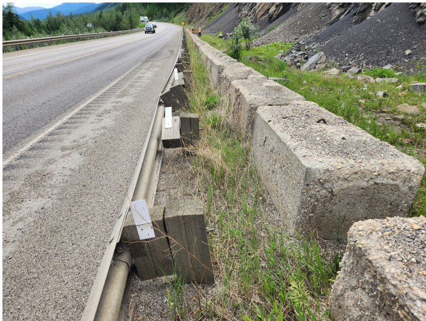
Photo 10 Segment of guardrail deflected and pushed towards southbound traffic from rockfall strike. Note lock blocks are deteriorating. Photo taken June 12, 2023, facing southwest.
