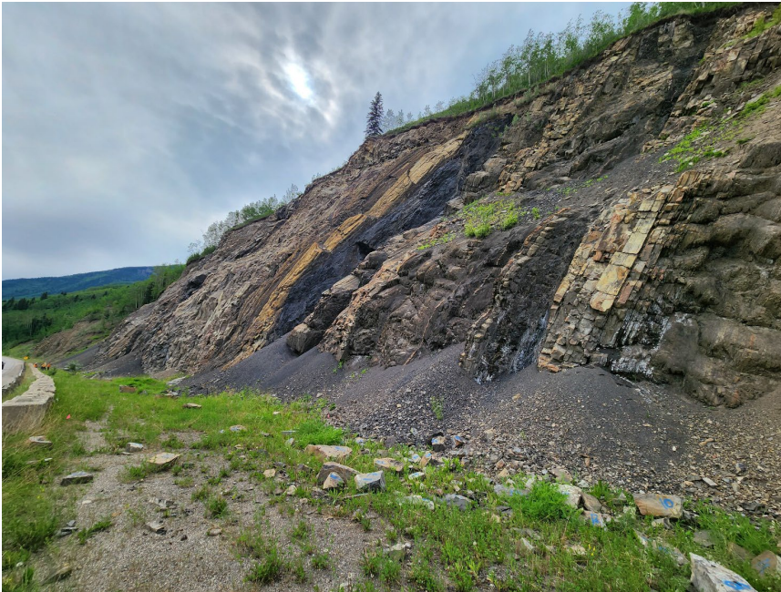
Photo 8 Rock slope along west side of Hwy 40:36 near northern site limit. Note hanging rock block (circled in white). Photo taken June 12, 2023, facing northwest.
