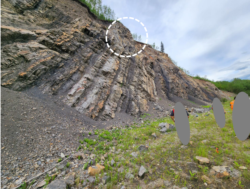
Photo 4 Potential rock block on upper slope shown in previous photo. Note dilated or open joints below rock block (indicated with white arrow), joints or shear planes to left and below rock block (circled in white), and rock and coal to right of rock block which is eroding. Photo taken June 12, 2023, facing northwest.
