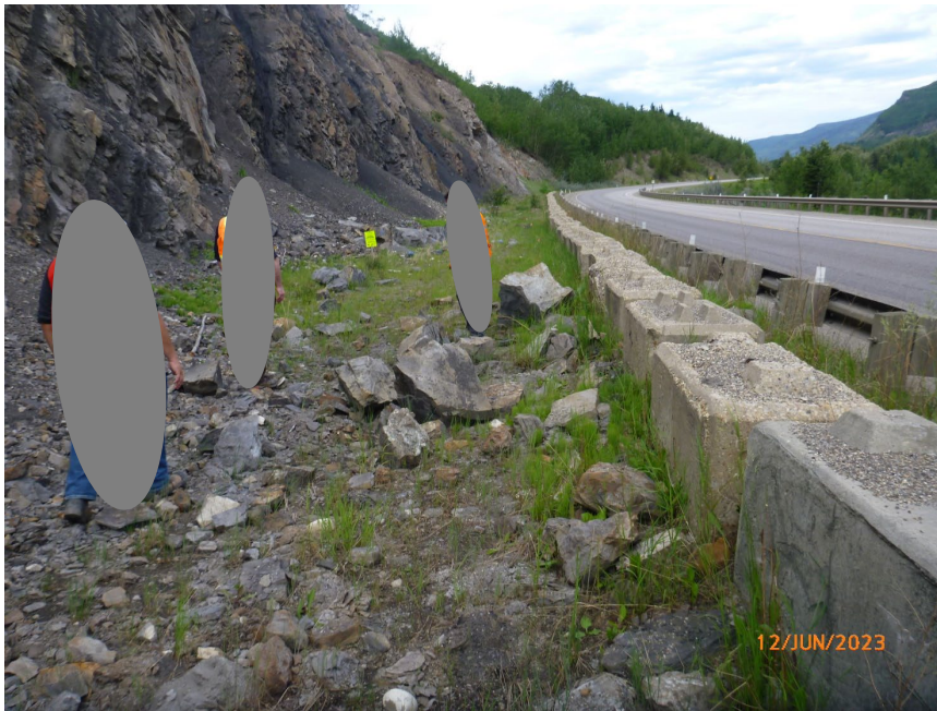
Photo 6 Rock slope along west side of Hwy 40:36. Note near-vertical bedding orientation of bedrock. Photo taken June 12, 2023, facing northwest.
