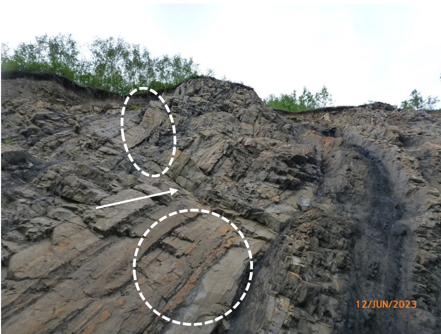
Photo 4 Potential rock block on upper slope shown in previous photo. Note dilated or open joints below rock block (indicated with white arrow), joints or shear planes to left and below rock block (circled in white), and rock and coal to right of rock block which is eroding. Photo taken June 12, 2023, facing northwest.
