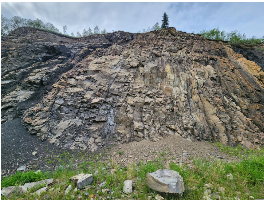
Photo 6 Rock slope along west side of Hwy 40:36. Note near-vertical bedding orientation of bedrock. Photo taken June 12, 2023, facing northwest.
