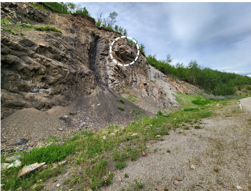
Photo 8 Rock slope along west side of Hwy 40:36 near northern site limit. Note hanging rock block (circled in white). Photo taken June 12, 2023, facing northwest.
