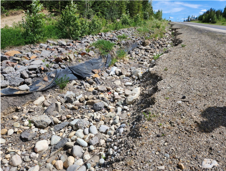
Photo 4 Erosion feature in north (westbound) ditch of Hwy 40:34 at WP295. Note recreational trail/road across erosion feature. Photo taken June 13, 2023, facing southeast.
