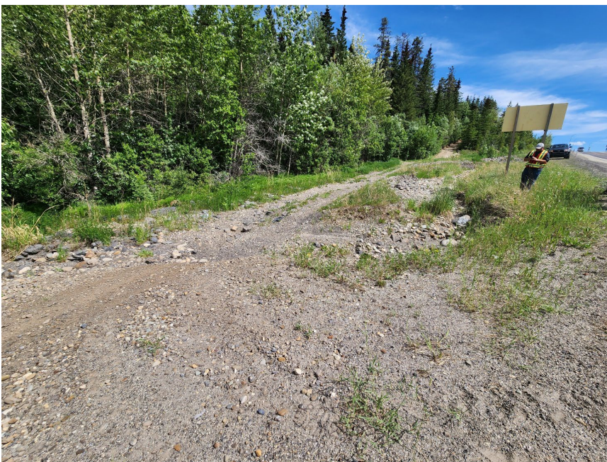
Photo 4 Erosion feature in north (westbound) ditch of Hwy 40:34 at WP295. Note recreational trail/road across erosion feature. Photo taken June 13, 2023, facing southeast.
