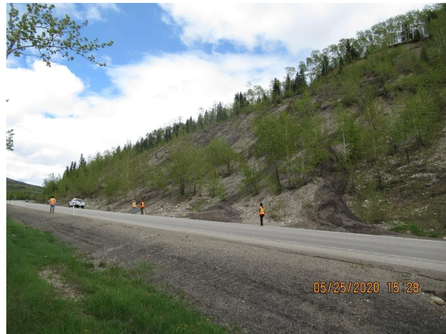
Photo 10. Looking northeast at backslope from across highway 40.
