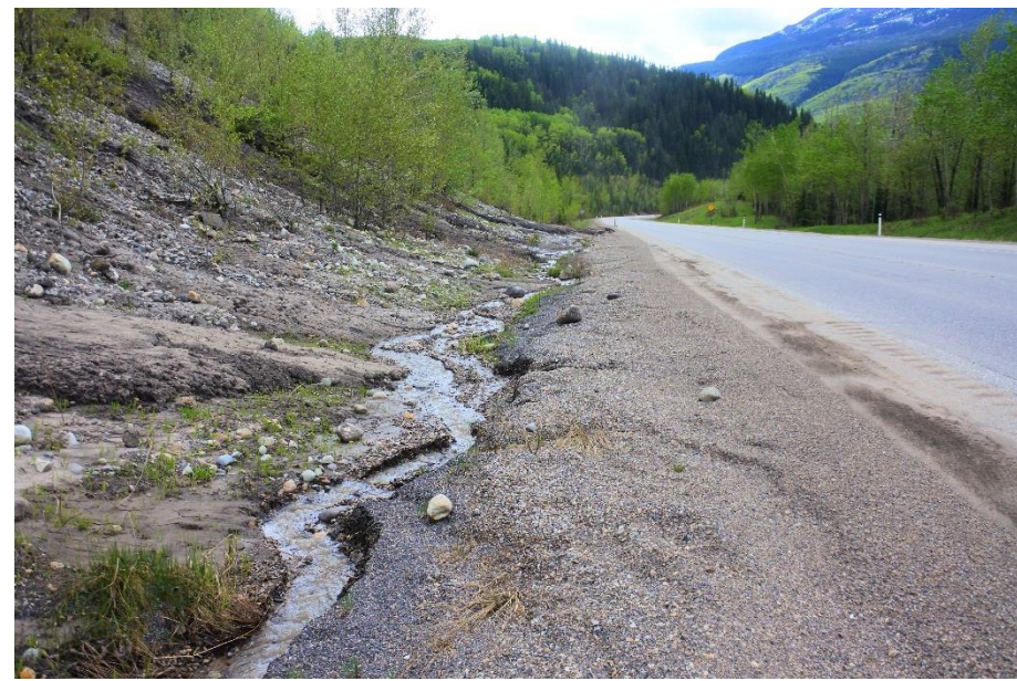
Photo 3. Looking southwest at east ditch and erosion that runoff is cutting down around the debris accumulation.
