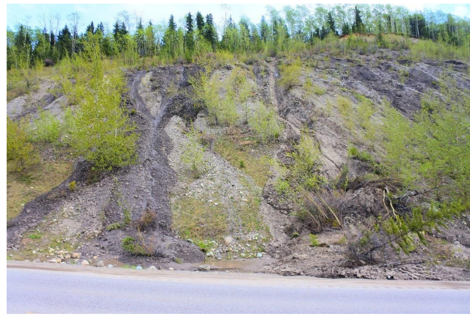
Photo 1. Looking southeast at shallow landslides/mudslide s down the backslope.
