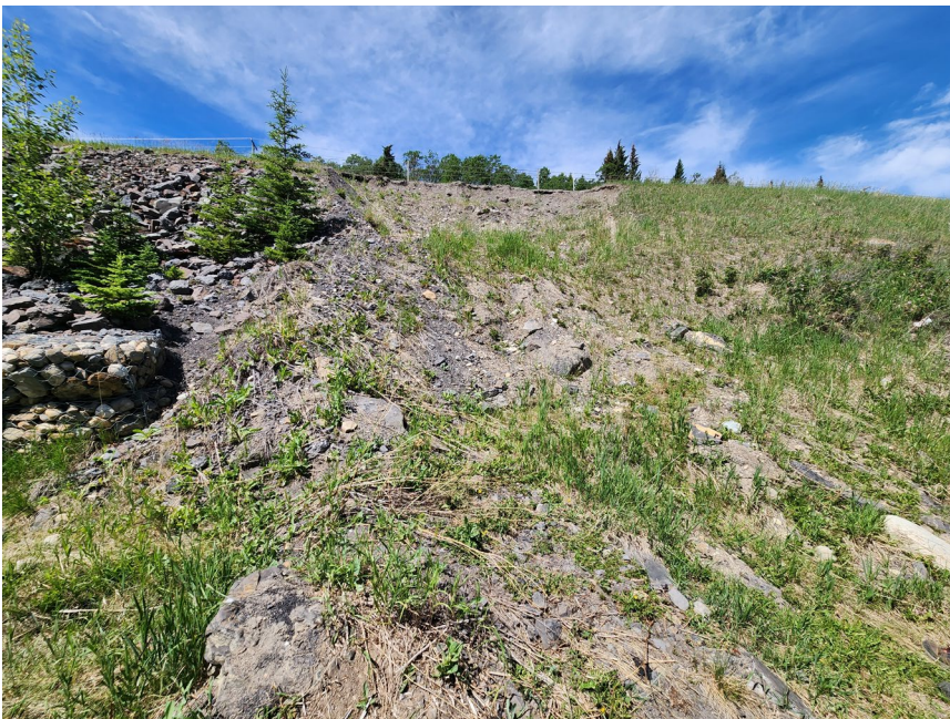
Photo 4 Slide and erosion area adjacent to previously repaired section on south side of Hwy 40:34. Photo taken June 13, 2023, facing northwest.
