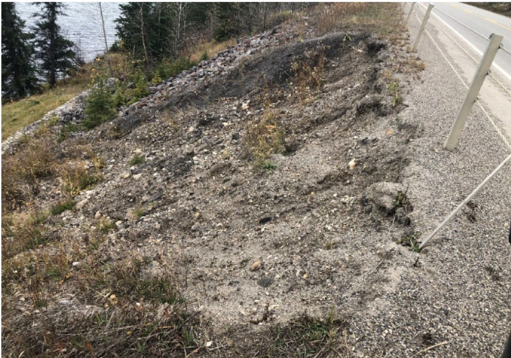
Photo 4 Crest of embankment slope near 2001 repair and recent failure. Photo taken on October 12, 2021, facing east.
