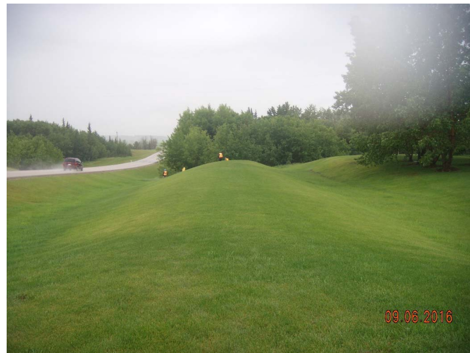
Photo 3. Looking south from private driveway at 130028 Hwy 724 along the berm west of SBL ditch.
