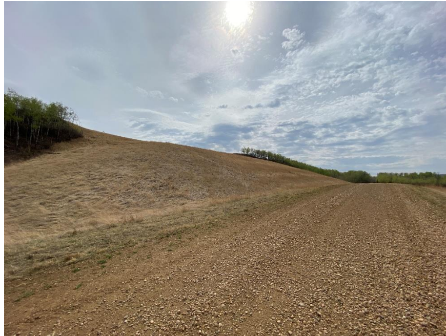
Photo 9. Looking southwest along the county road on the toe berm.
