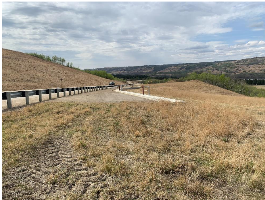
Photo 2. Looking west at pile wall alignment.
