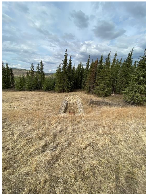
Photo 10. Looking north at drop pipe outlet.
