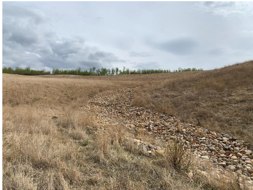
Photo 6. Looking northwest at west riprap channel.
