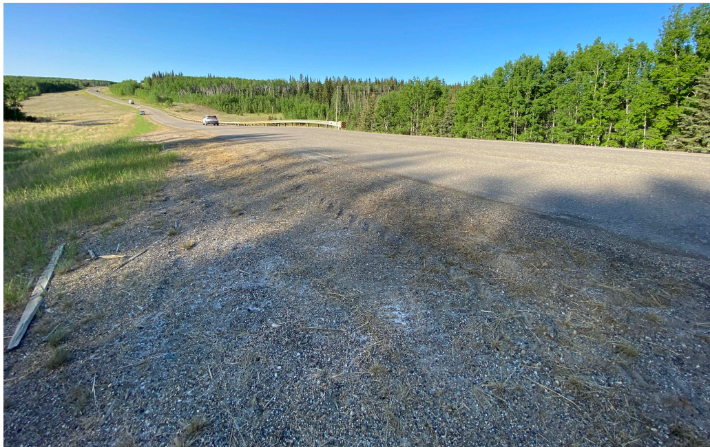
Photo 8 - Looking south along the highway from the south end of the scarp of Site 5.
