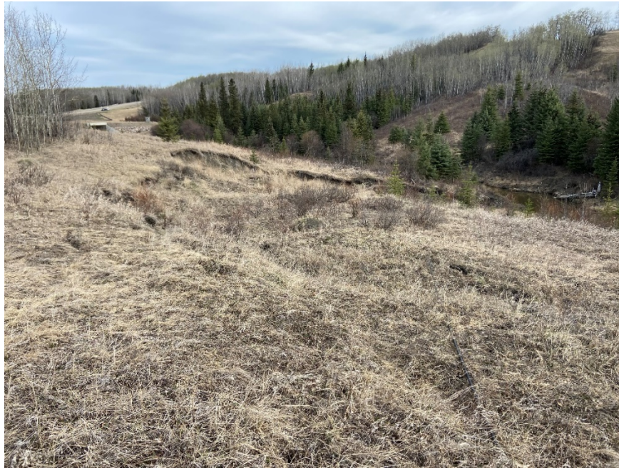
Photo 5 – Looking north along the east highway embankment from the south end of Slide Site 2.
