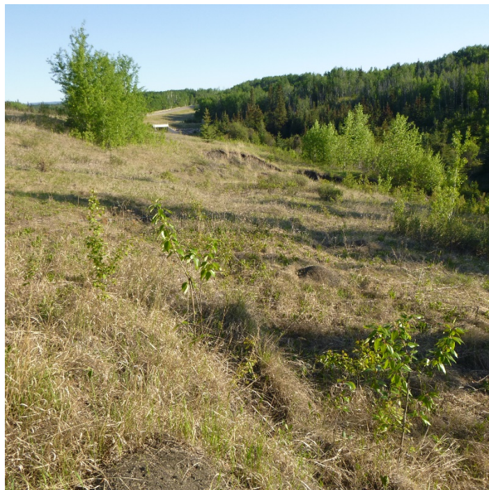
Photo 4 – Looking north along the east highway embankment from the south end of Slide Site 2.
