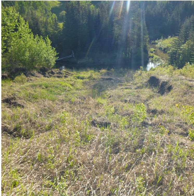
Photo 5 – Looking southeast at the outside bend of the river, which is causing the most active slumping area at Site 2.
