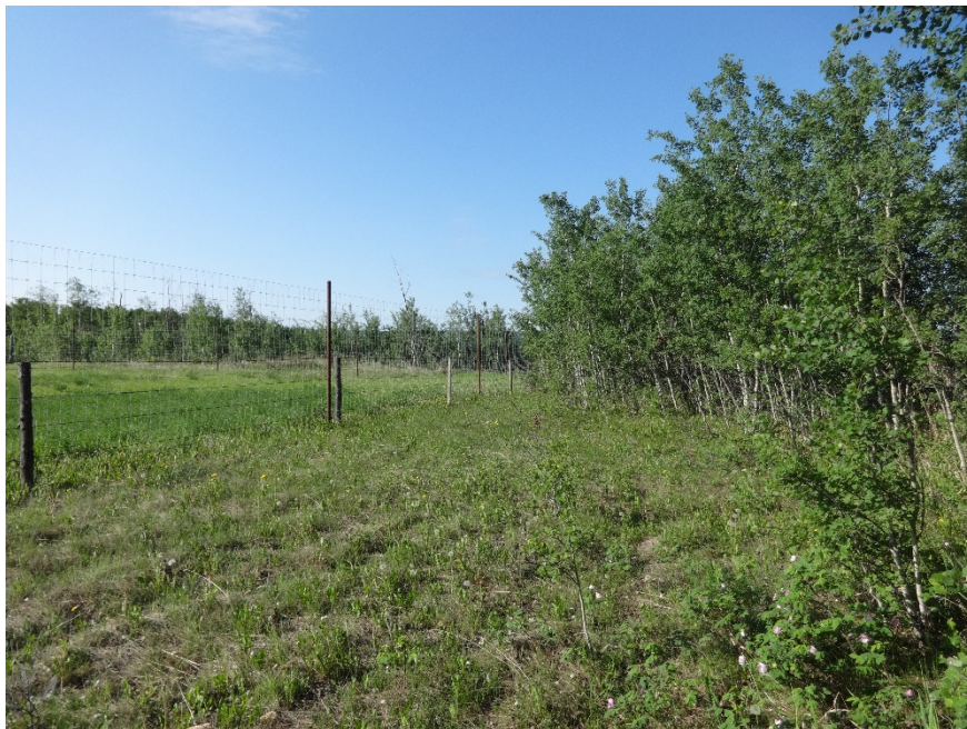
Photo 6. Looking south at farm fence above the slope failure. Photo credit: Nicole Wilder.
