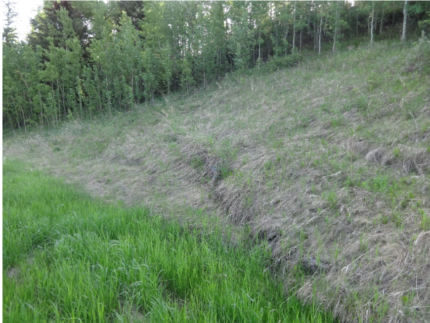
Photo 5. Looking northeast at where noticeable toe roll is. Photo credit: Nicole Wilder.
