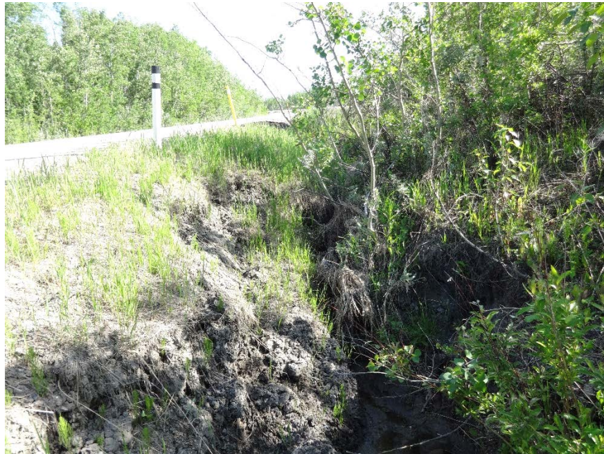
Photo 11. Looking north at erosion gully just south of where pavement was affected. Photo credit: Nicole Wilder.
