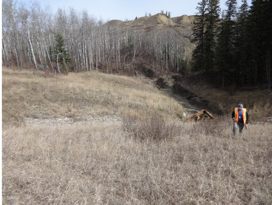
Photo 13. Looking north at eroded tributary channel, trash rack and upstream slope instabilities north of the highway at PH077-2. Photo Credit: Nicole Wilder.
