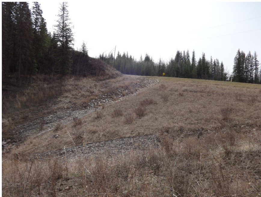
Photo 10. Looking southeast at the v-shaped ditches on the north side of the highway. Photo Credit: Nicole Wilder.
