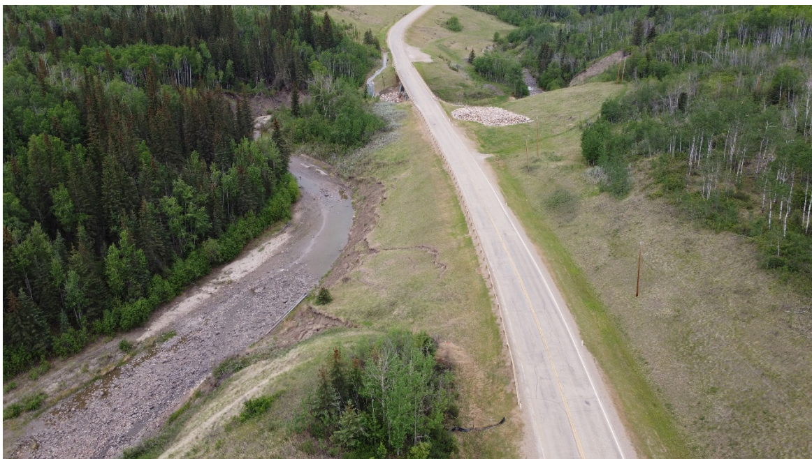
Photo 16. Looking northwest at PH077-2. Drone Photo Credit: Don Proudfoot.
