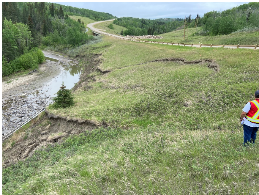
Photo 5. Looking west at new slump that developed west of the knob hill. Photo Credit: Don Proudfoot.
