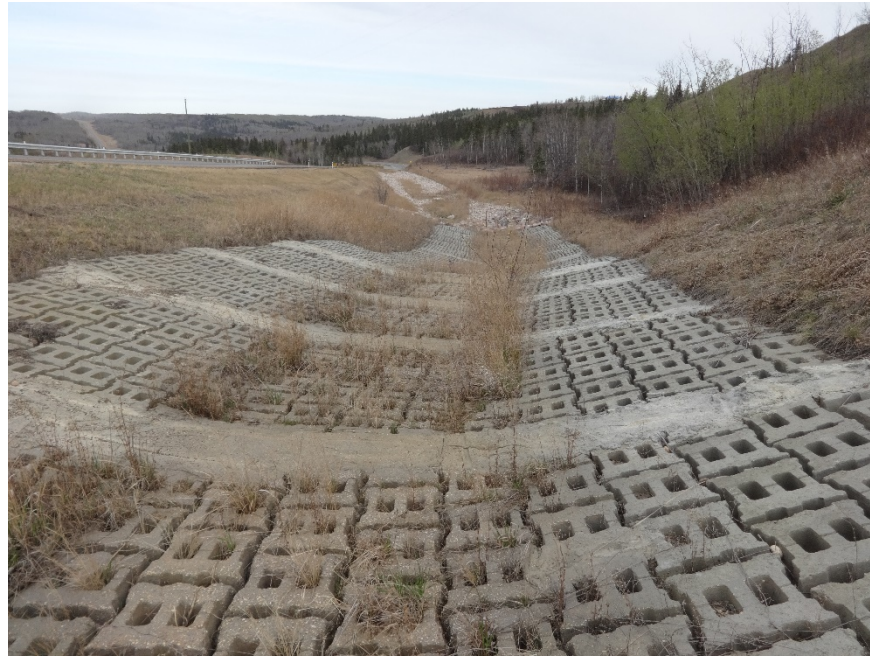
Photo 11. Looking northwest at the ACB Matting that was previously grouted. Photo Credit: Nicole Wilder.
