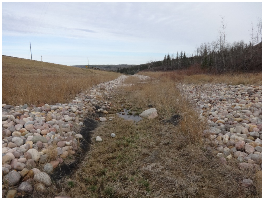
Photo 10. Looking east at area within riprap that now has mud and grass covering some of the riprap likely from high runoff flow events and ponding afterwards. Photo Credit: Nicole Wilder.
