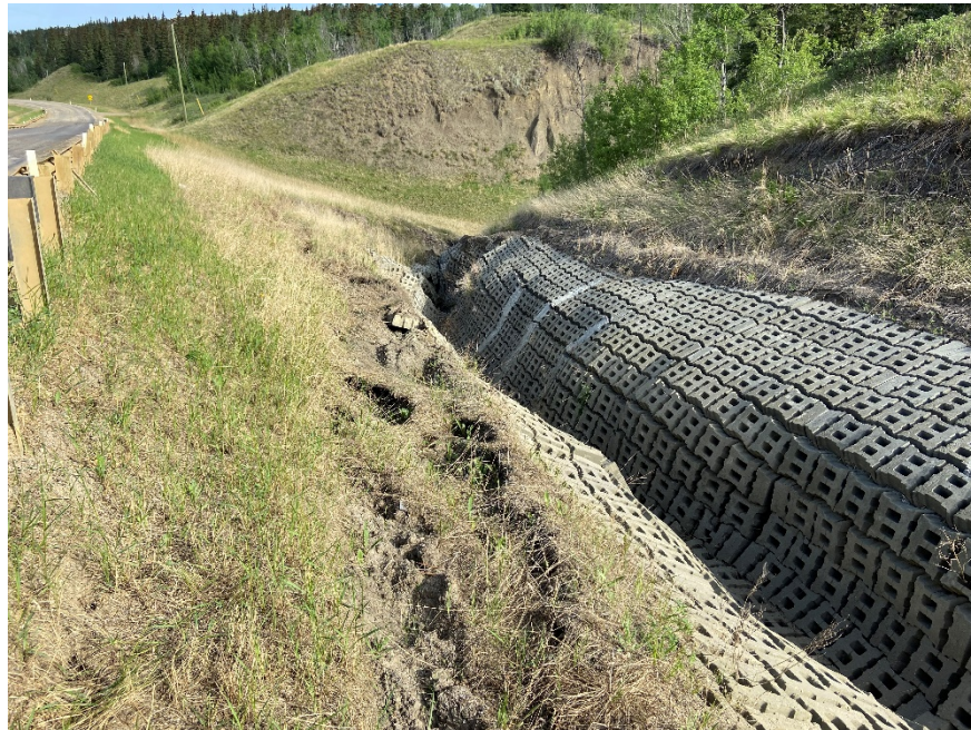
Photo 3. Looking northwest along the severely damaged ACB mat area and enlarged slide scarp area. Photo credit: Don Proudfoot.
