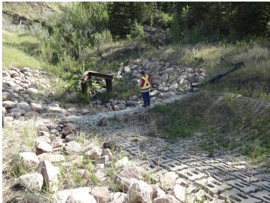
Photo 7. Looking northwest across the eroded mat area near the bottom of the slope. Photo Credit: Don Proudfoot.
