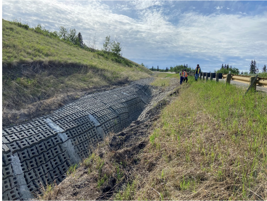
Photo 1. Looking east along the beginning of the eroded ACB mat area north of the highway. Photo credit: Nicole Wilder.
