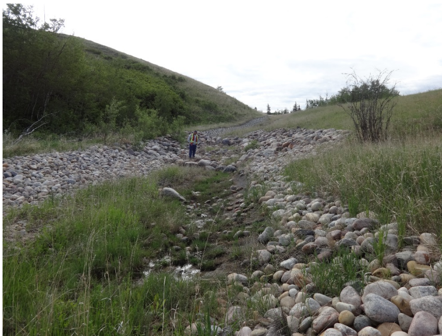
Photo 13. Looking east at area within riprap that now has mud covering some of the riprap likely from high runoff flow events and ponding afterwards. Photo Credit: Nicole Wilder.
