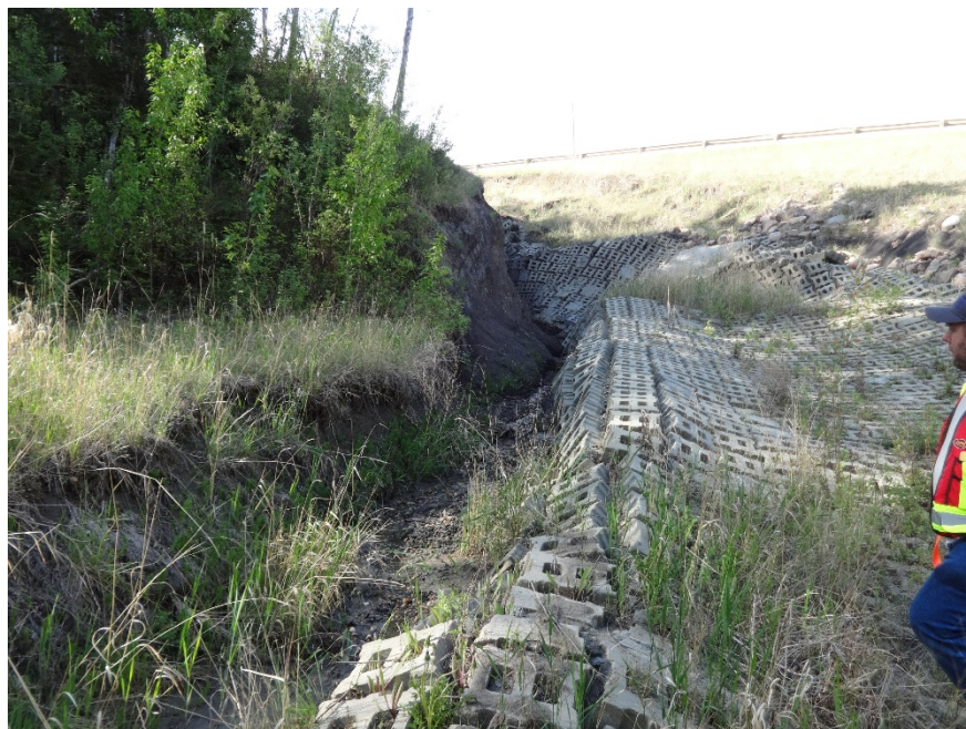
Photo 5. Looking southeast along the north edge of the eroded ACB mats. Here the mats have slid down into the deeply eroded channel, exposing the underlying gravel. Photo Credit: Nicole Wilder.
