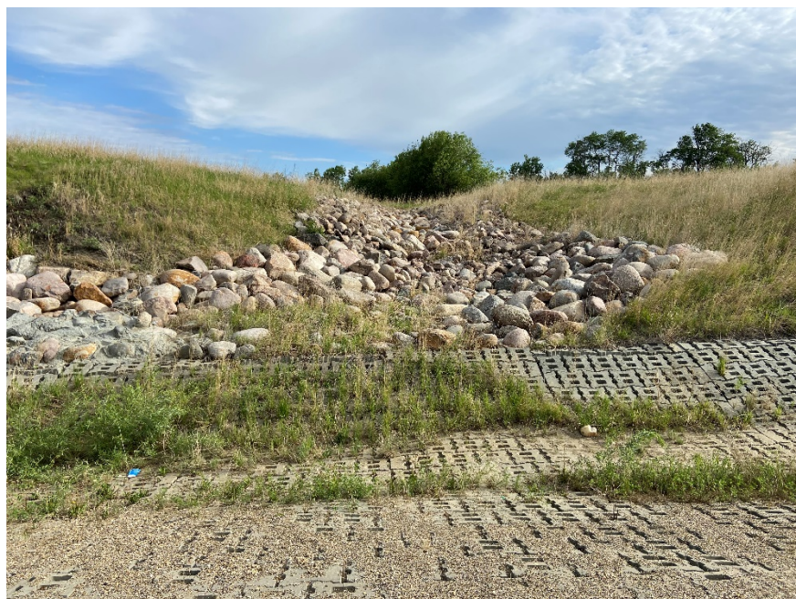
Photo 12. Looking north at where riprap was previously placed, appears to be in good condition. Photo Credit: Don Proudfoot.
