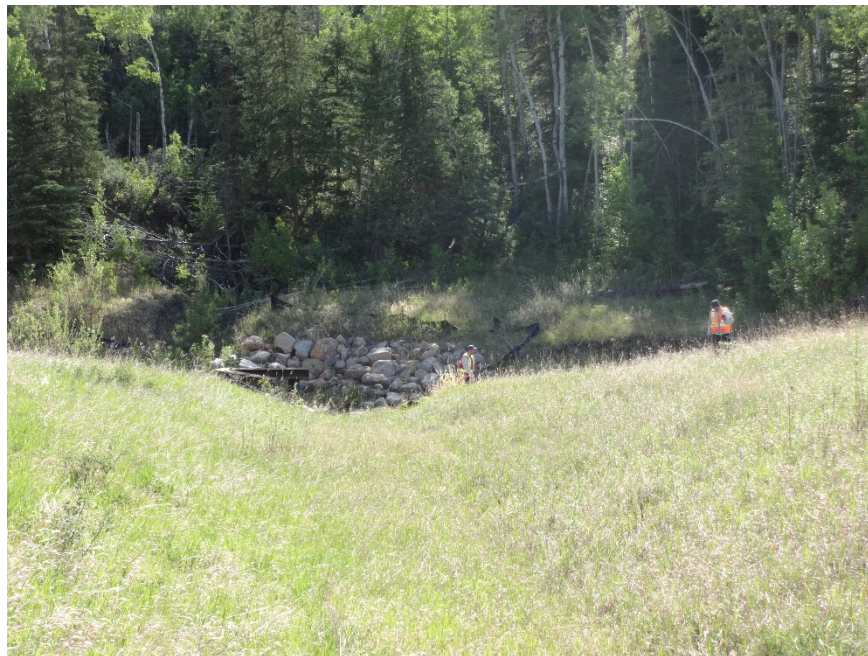
Photo 9. Looking north at the slumping and infill occurring into the channel upstream of the 1524 SWSP culvert entrance. Photo Credit: Nicole Wilder.
