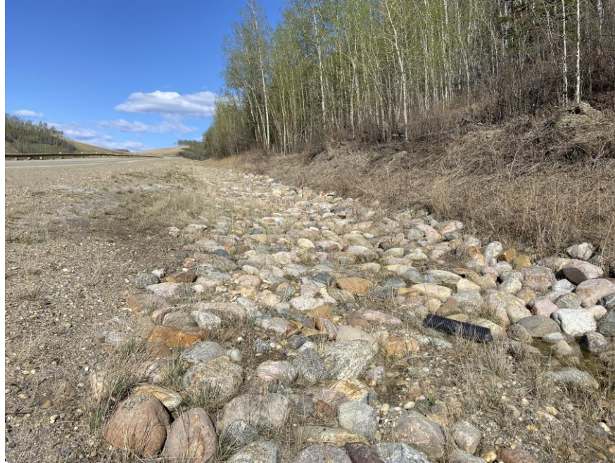
Photo 3 – Looking east from near the ditch block along the riprapped south ditch channel from just upslope of the inlet of the 760 mm dia. SWSP.
