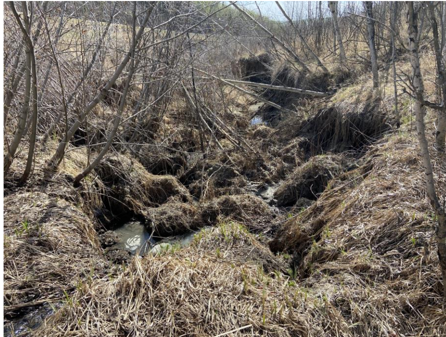
Photo 15 – Looking west (downstream) at the erosion just upstream of the 760 SWSP outlet.
