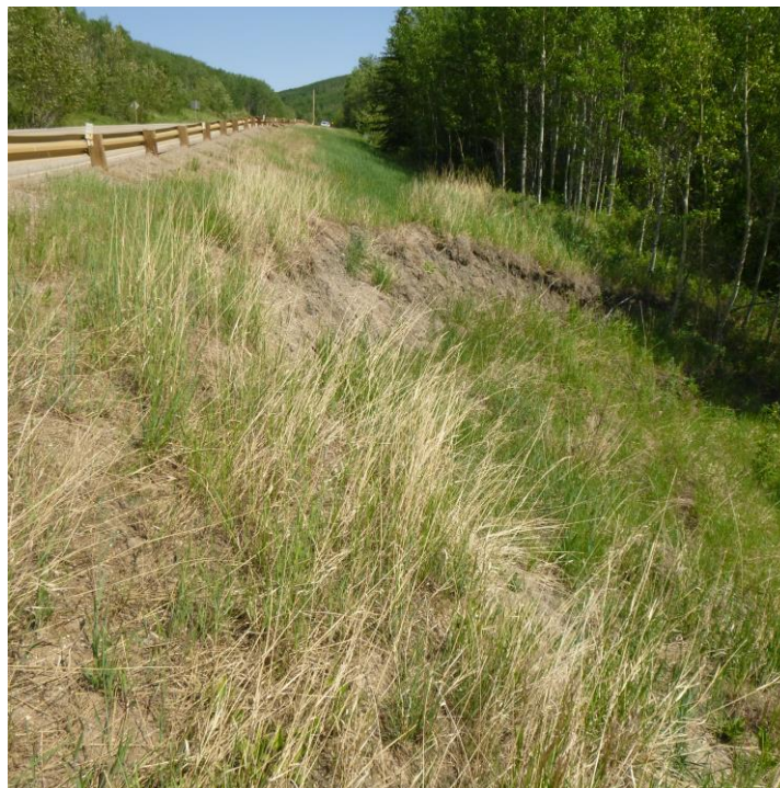
Photo 4 – Looking east at Embankment Slump A on the south side of the hwy.
