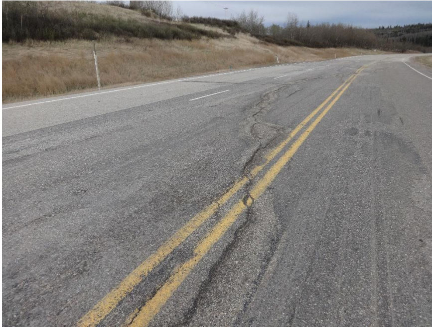
Photo 9. Looking east from near the middle of the 2021 ACP patch where crack continues into WBL. Photo Credit: Nicole Wilder.
