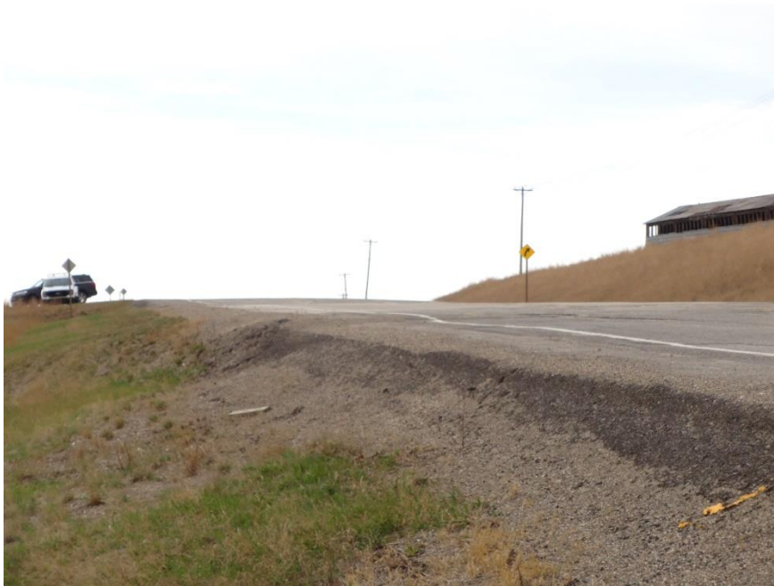
Photo 14. Looking north at the thick accumulation of asphalt patches in the landslide area . Photo Credit: Nicole Wilder.
