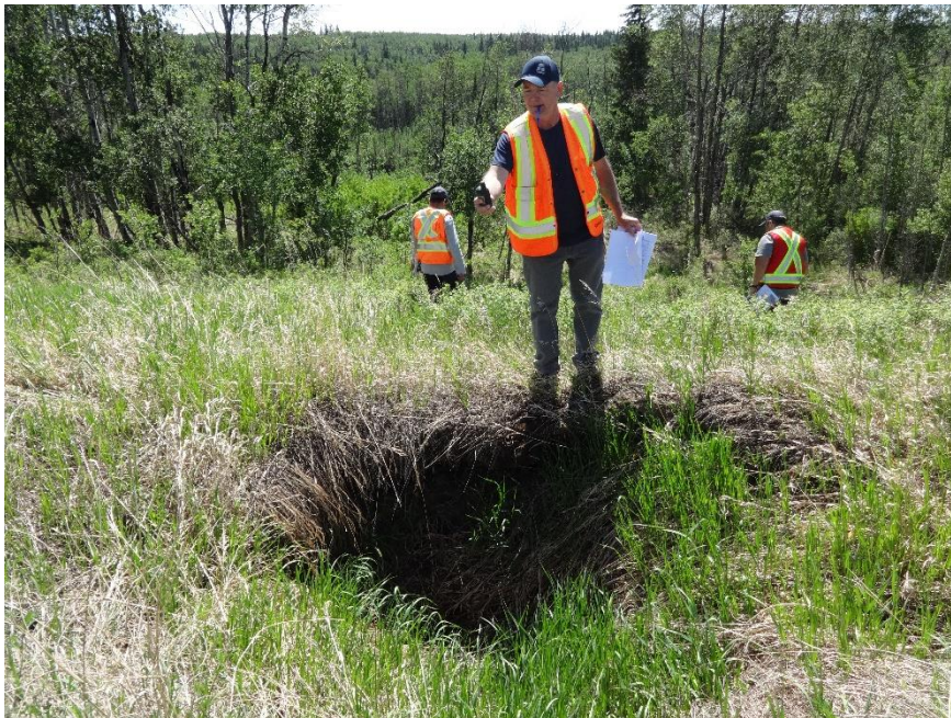
Photo 14. Looking south at 1.5 m diameter sinkhole. Photo Credit: Nicole Wilder.
