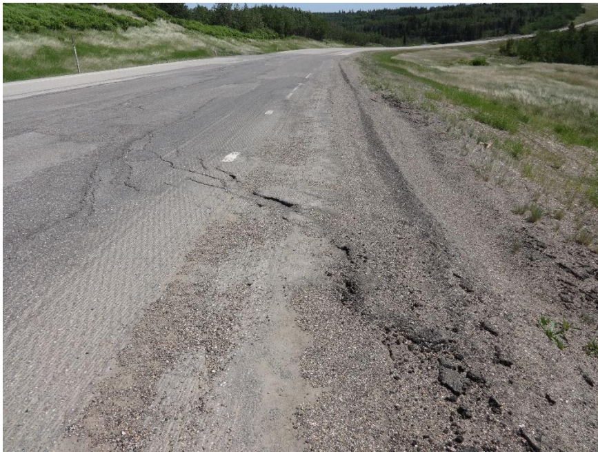
Photo 6. Looking east from the shoulder of the EBL of Hwy 49:06 at the westmost dip in the 2021 ACP patch. Photo Credit: Nicole Wilder.
