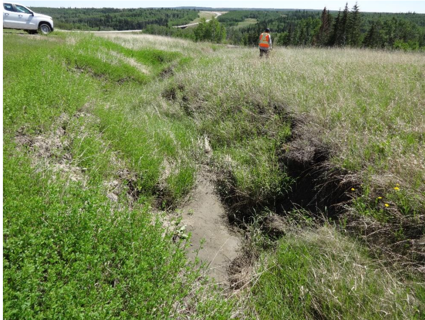
Photo 1. Looking southeast at erosion gully that had formed in the south ditch which had pooling water in it in 2022 but only some of the scour holes had water in 2023. Photo credit: Nicole Wilder.
