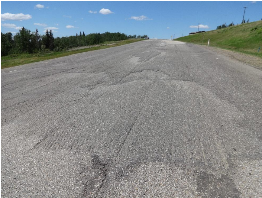
Photo 10. Looking northwest from the EBL of Hwy 49:06 at the south end of the site. Photo Credit: Nicole Wilder.
