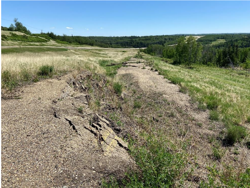
Photo 3. Looking southeast at where scarp crosses the old highway alignment. Photo credit: Don Proudfoot.
