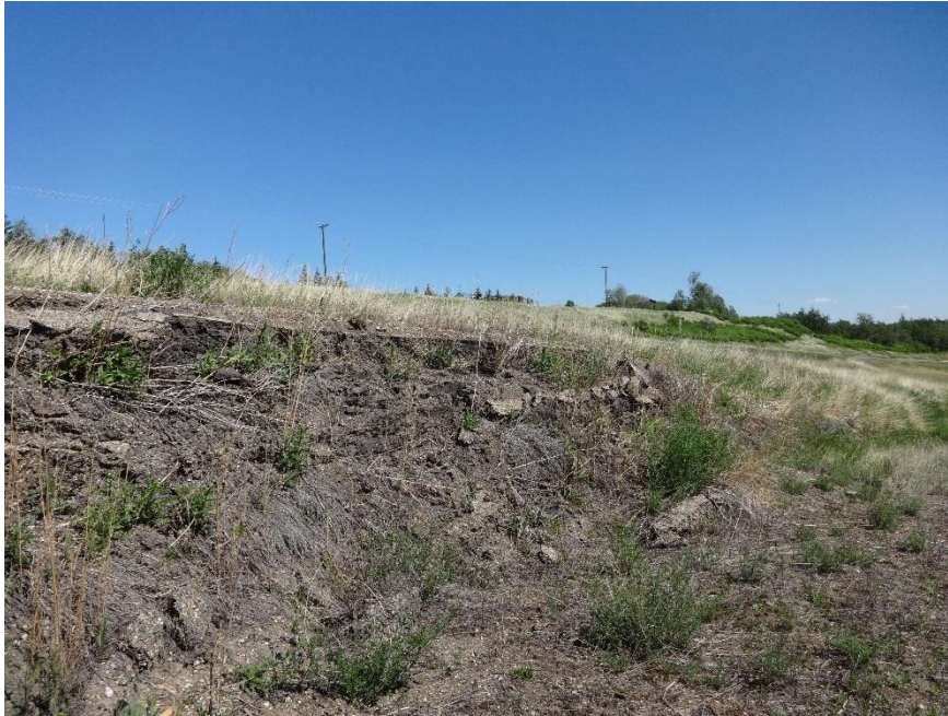
Photo 5. Looking southeast from old highway alignment at south slide scarp. Photo Credit: Nicole Wilder.
