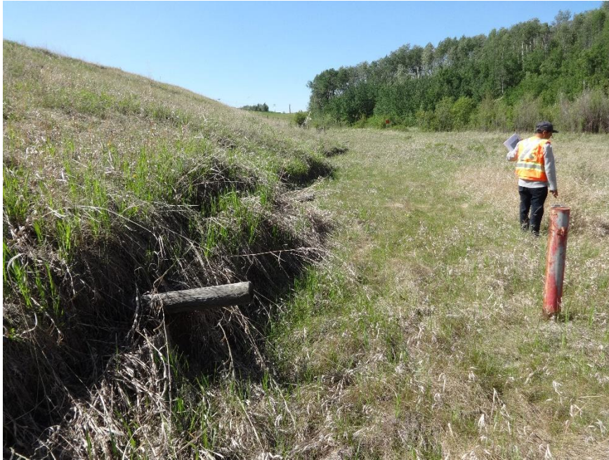
Photo 5. Looking northwest along the toe of the landslide. The fence posts are bent over further from movement of the toe bulge. Photo Credit: Nicole Wilder.
