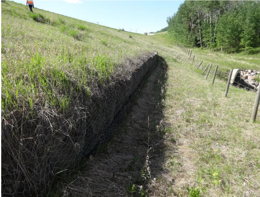
Photo 7. Looking northwest along the gabion wall. Photo Credit: Don Proudfoot.
