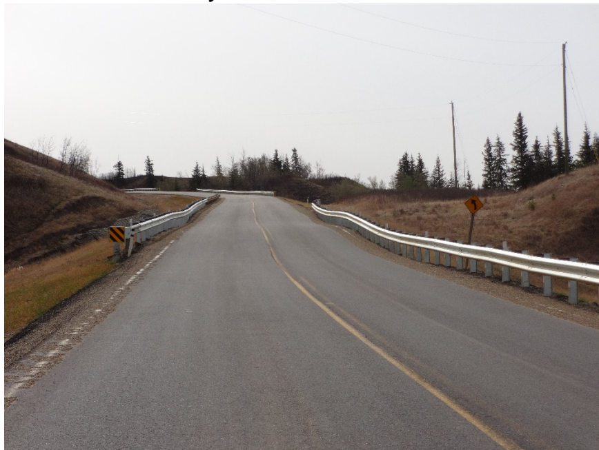
Photo 4. Looking east along the highway at where it was paved but you can see the dip in the guardrail. Photo credit: Don Proudfoot.
