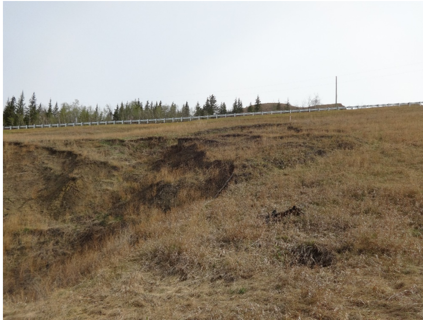
Photo 5. Looking northwest towards the landslide and backscarp. Photo Credit: Don Proudfoot.
