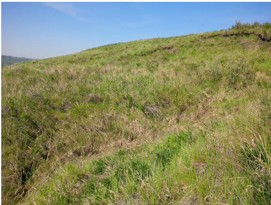
Photo 12. Looking northwest at large backscarps forming at the crest of the valley slope.
