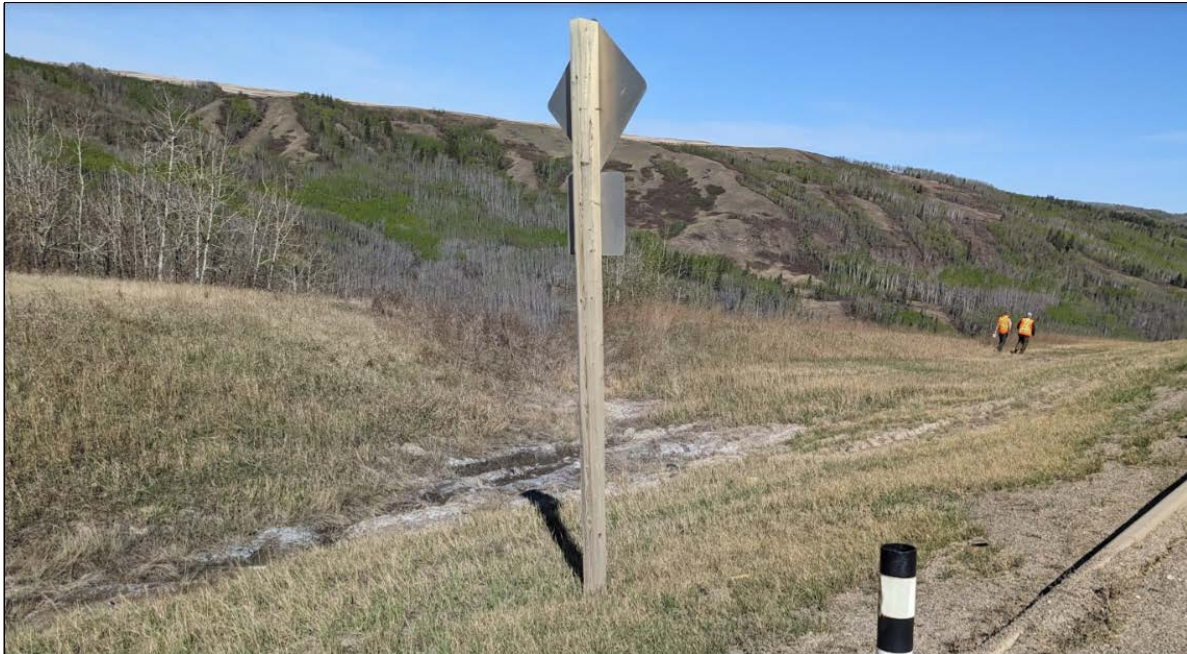
Photo 1: Looking northwest from Sta. 2+000 at erosion gully in SBL ditch south of ditch block
