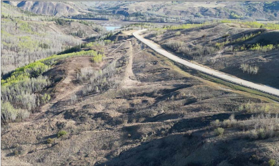
Photo 17: Oblique Drone Photo looking at overall site showing slumps along the highway sideslope
