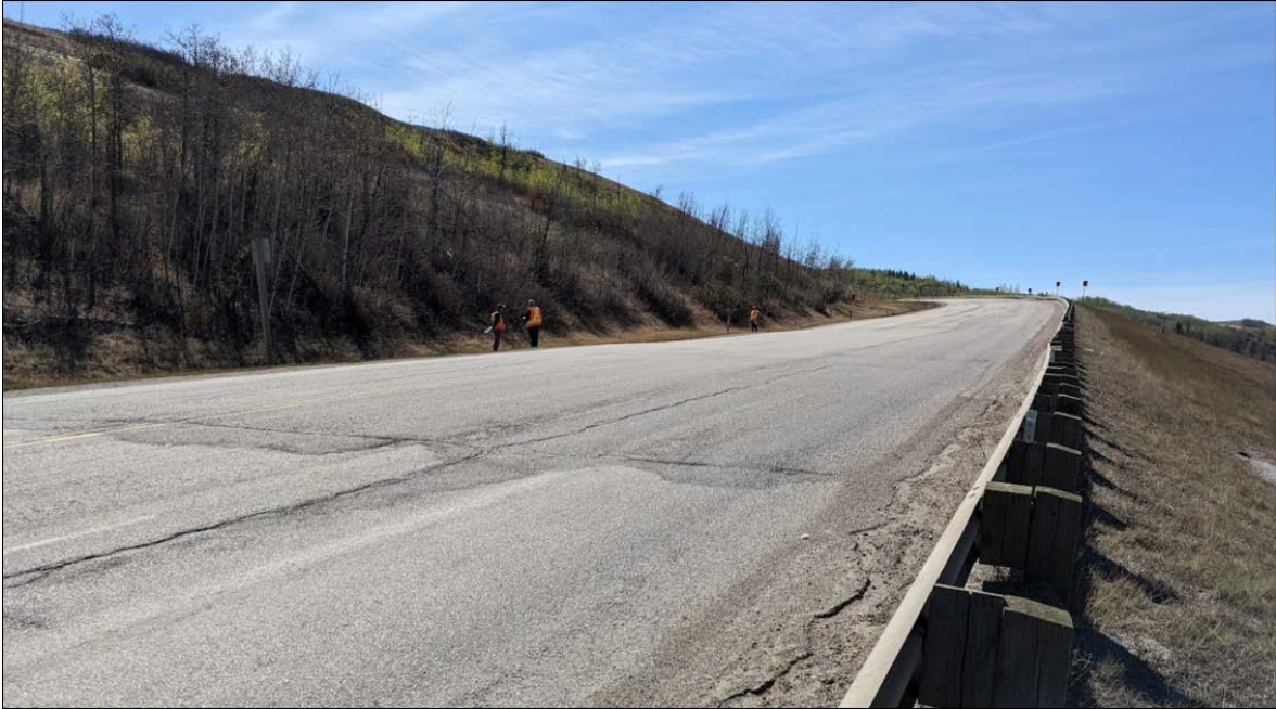
Photo 7: Looking from the shoulder of the SBL at Sta. 1+670 across the dip in the highway at the north end of the 1+800 slide.
