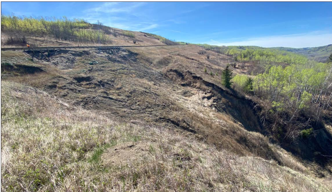
Photo 14: Looking south towards the 1+400 slide. The slide has further retrogressed towards the highway, is wider than in 2023 and there is a 5 m to 7.5 m drop below the guardrail.
