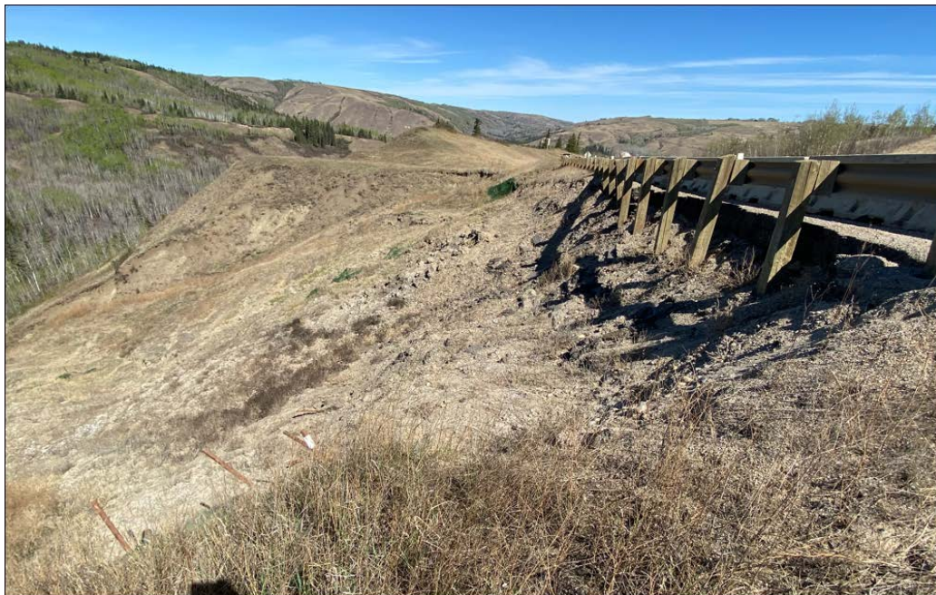
Photo 12: Looking north from Sta. 1+450 backscarp.
