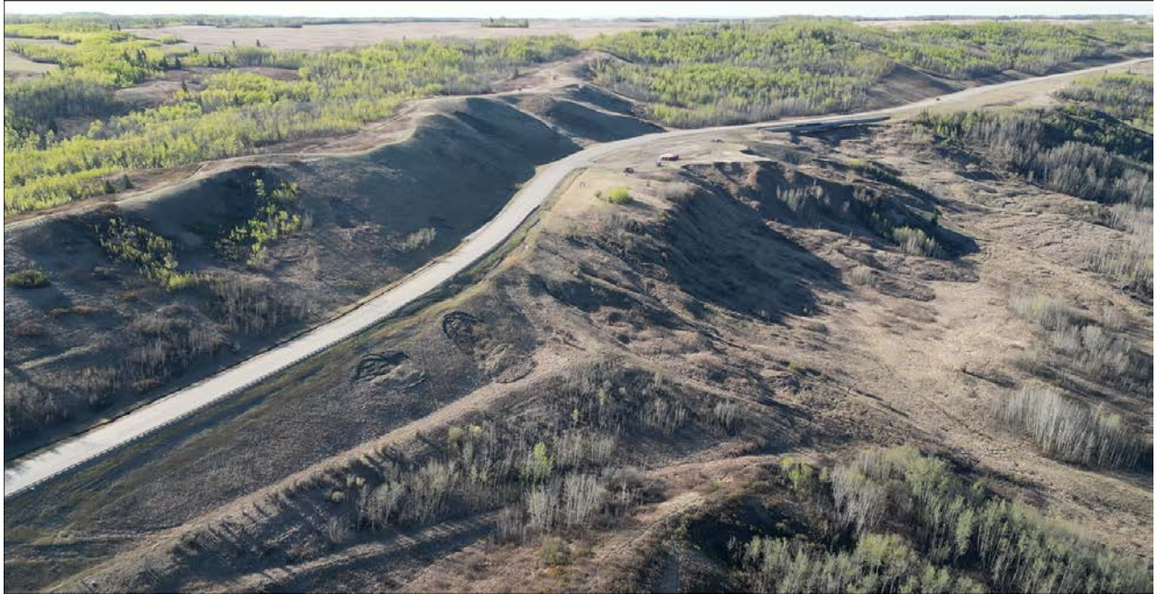
Photo 19: Oblique Drone Photo looking at south half of the site showing backslope slumps located north of Pile Wall at PH035
