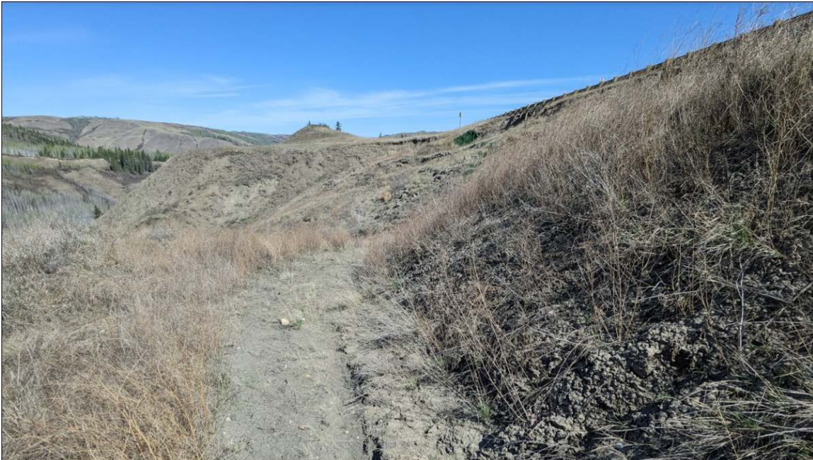
Photo 16: Looking north at slumping occurring from Sta. 1+450 to 1+550. Photo showing a drop of about 0.1 m.
