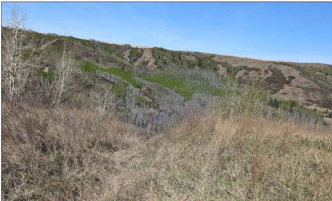
Photo 2: Looking west from Sta. 1+980 below the SBL highway. More movement noted in 2024
