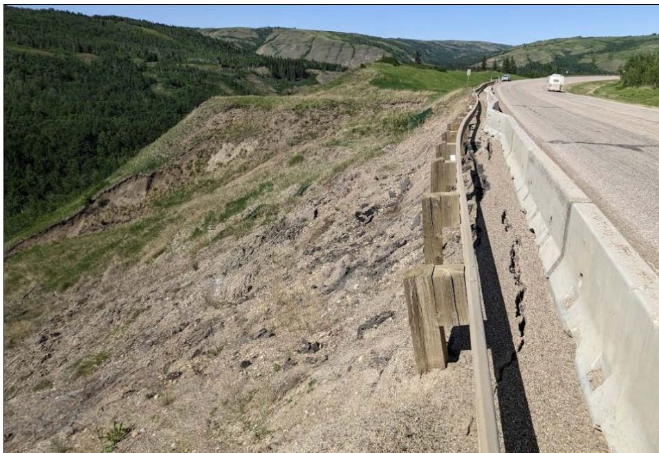
Photo 12: Looking north from Sta. 1+450 backscarp. New Jersey Barrier installed in 2023
