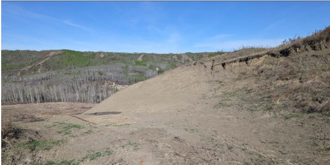
Photo 3. Looking at graded Borrow Area B used during the 2023 repairs.
