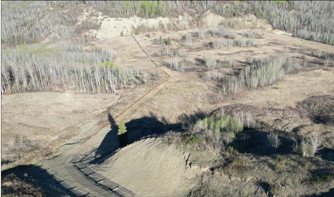
Photo D1. Oblique drone view of elephant trunk on lower slope
