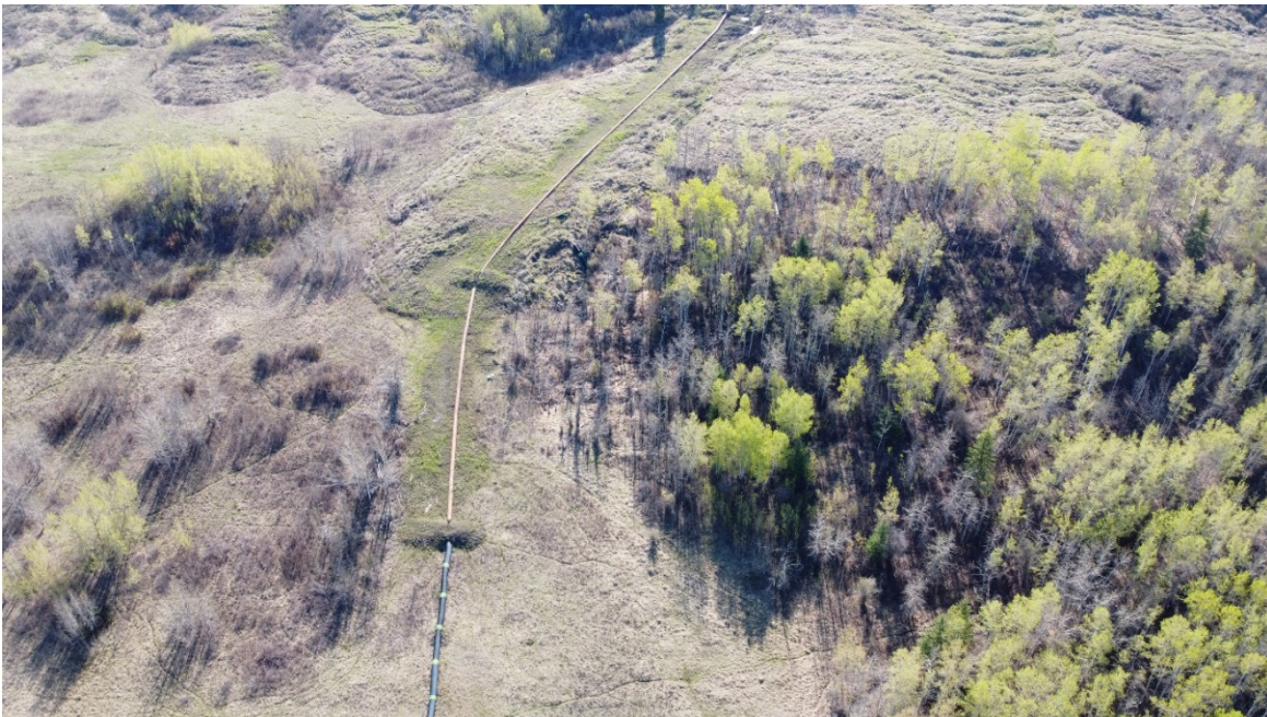
Photo D4. Oblique drone view of elephant trunk on lower slope
