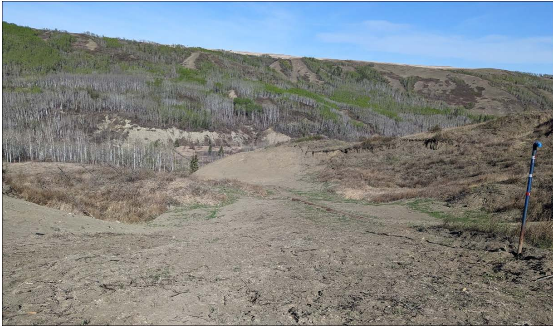
Photo 1. Looking northeast from Sta. 2+320 towards the Dunvegan Elephant Trunk consisting of a 760 mm diameter smooth wall steel pipe
