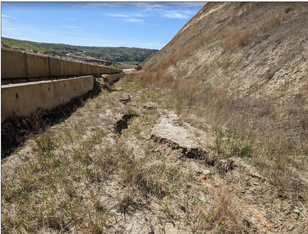
Photo 4: Area where sandstone slabs, talus, boulders accumulated the most prior to the 2022 clean up.
