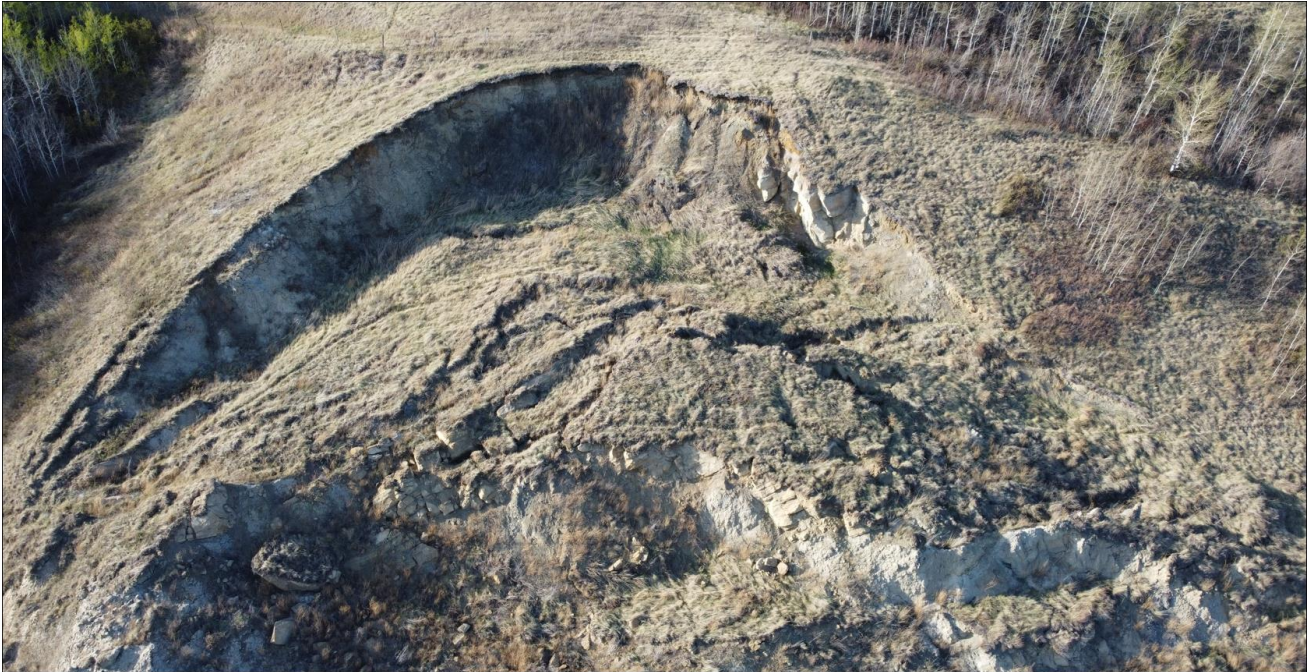
Aerial Photo 5: Looking northwest where landslide debris has been toppling over the edge of the steep bedrock slope
