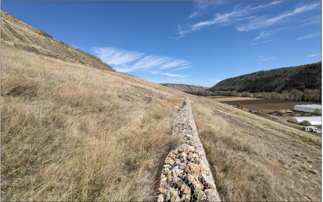
Photo 11: Gabion Basket. Acceptable condition in 2024
