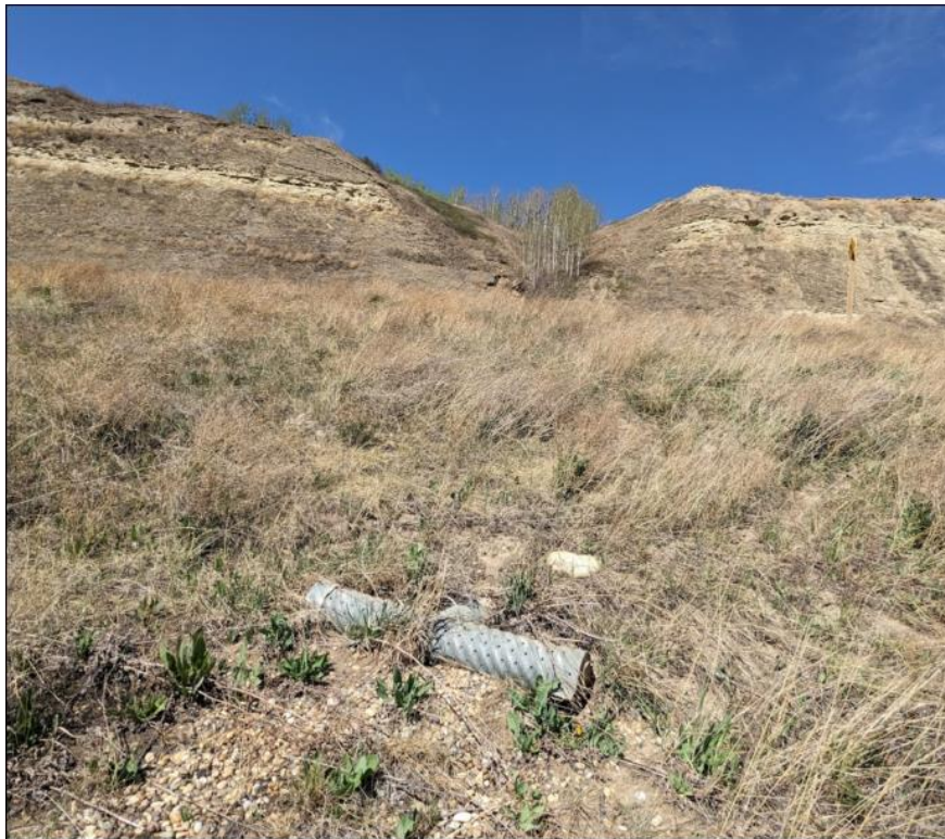
Photo 9: Subdrain outlet located upslope from gabion basket. Dry in 2024
