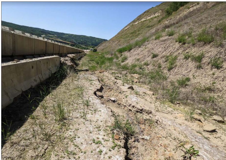
Photo 4: Area where sandstone slabs, talus, boulders accumulated the most prior to the 2022 clean up.
