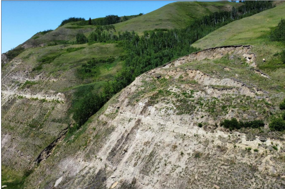
Aerial Photo 9: Note graben formed along the backscarp, sandstone rock slabs resting on the slope near the bottom, and seepage in the central area developing near the toe of the slide.
