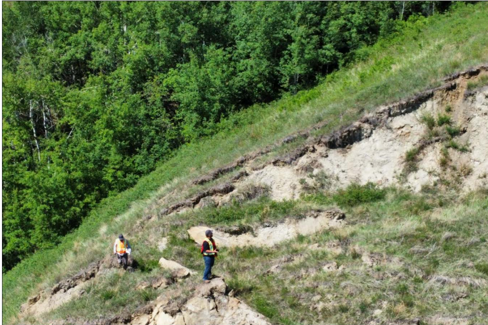
Aerial Photo 7: Looking west landslide backscarp western flank
