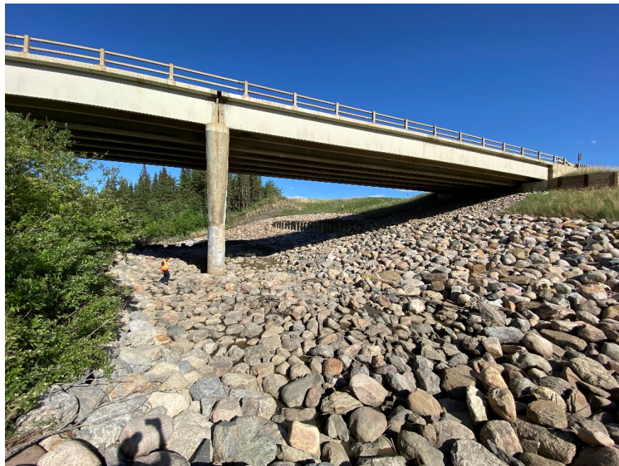
Photo 9. Looking southeast at the pier and riprap. Photo Credit: Nicole Wilder.
