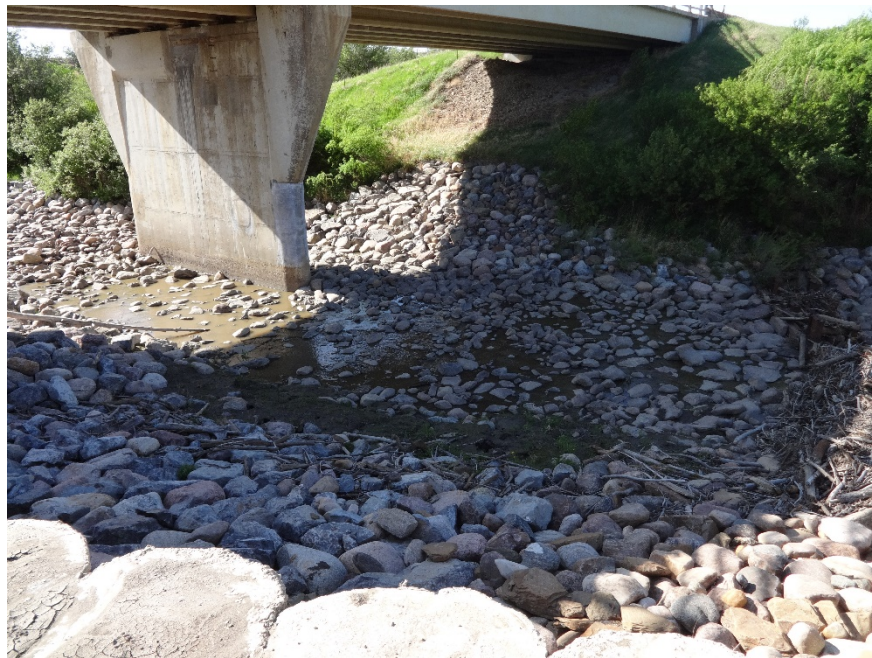
Photo 11. Looking northwest at the north head slope. Photo Credit: Nicole Wilder.
