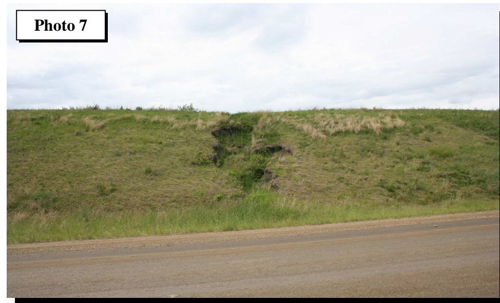
Looking west (another view) - Erosion gully at backslope at upper portion of river valley
