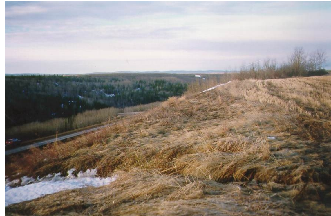
Photo 14 Looking south downgrade (along top of valley slope edge of upland farm area) 1) Surface water outfall down backslope to cause concentrated flow erosion 2) No swale or catchwater ditch (dyke) along perimeter of upland farm
