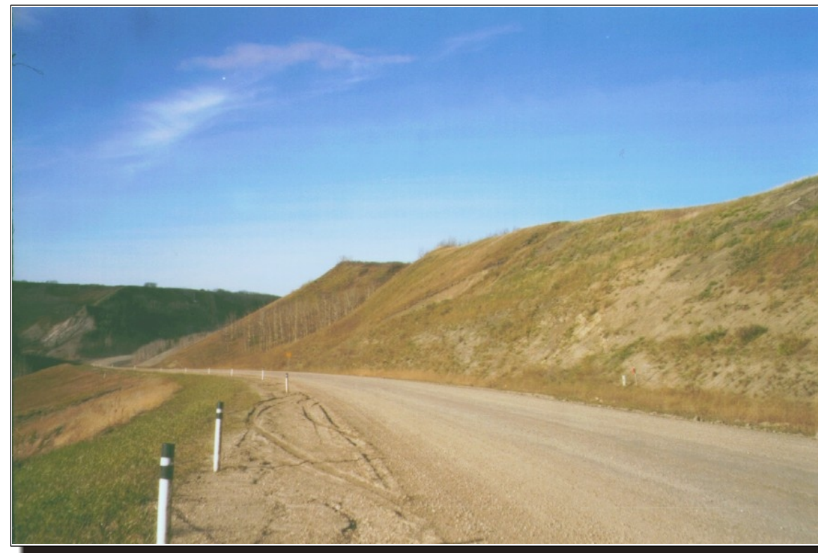
Photo 3c Looking downgrade. Steep backslope as result of previous alignment shifts towards upland.
