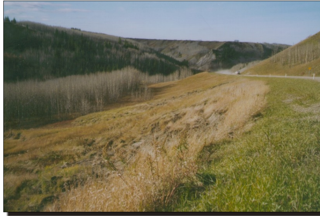
Photo 5a Slides along sideslope.
