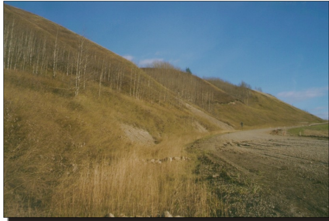
Photo 5e Another view of slide headscarp crossing highway and backslope.
