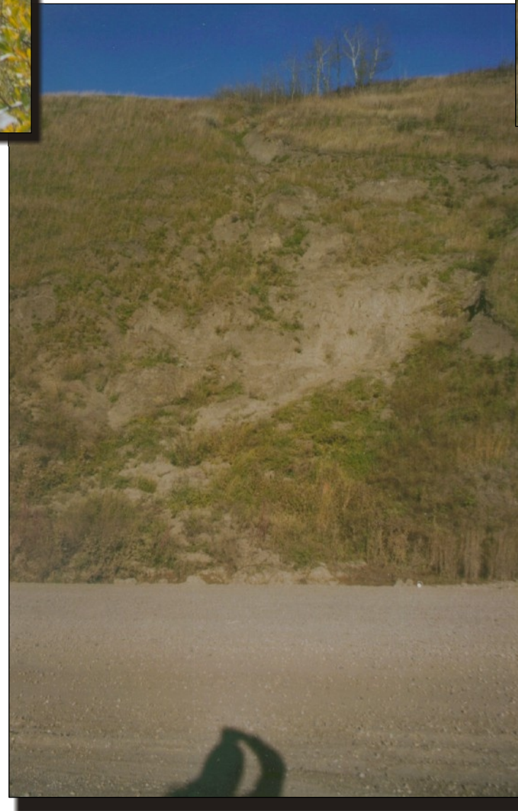
Photo 4b Looking upslope. Erosion slide of backslope.
