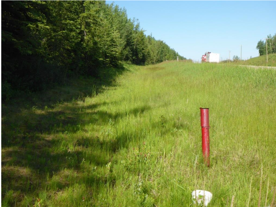
Photo 5: Well vegetated toe bulge south of SI01-1. Looking west.
