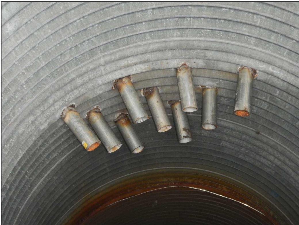
Photo 3: East drainage gallery – zero of nine running
