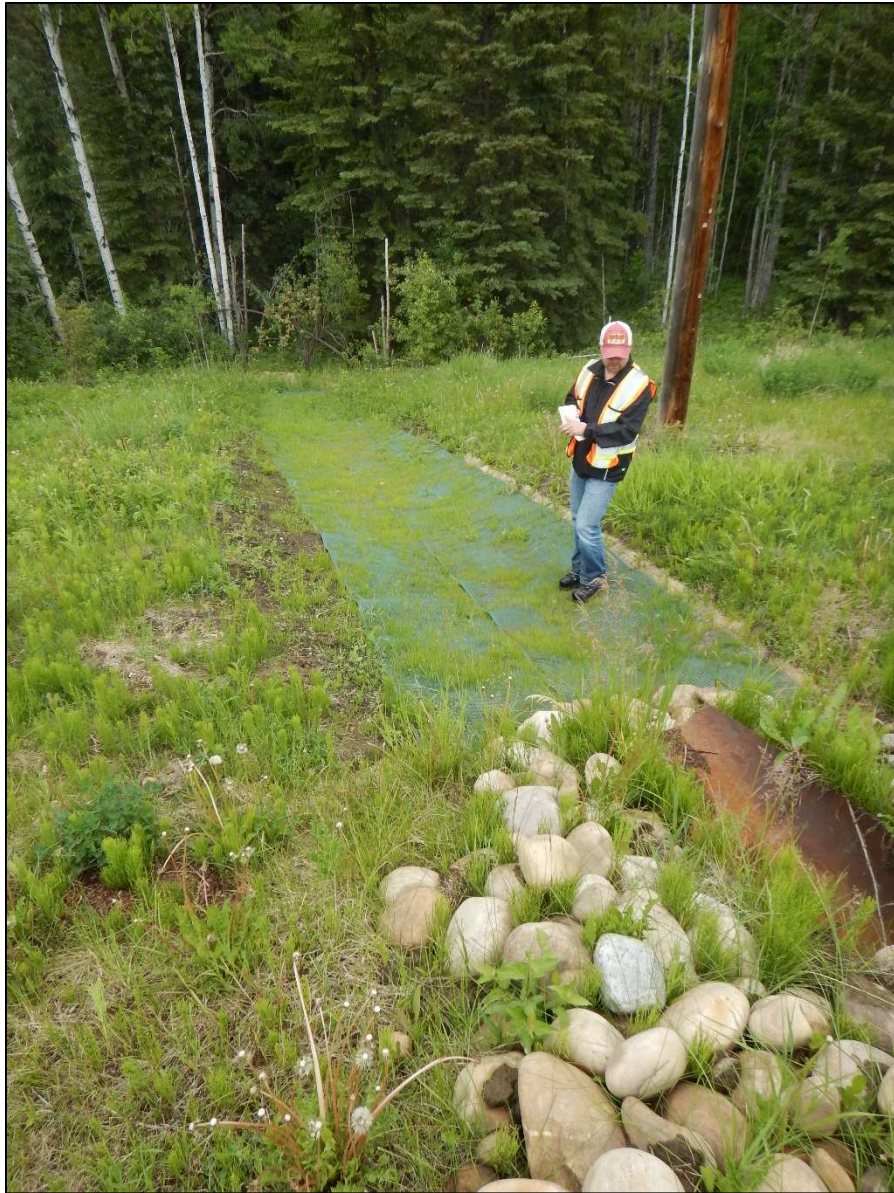
Photo 1: Recently installed erosion and sediment control at outlet of east culvert
