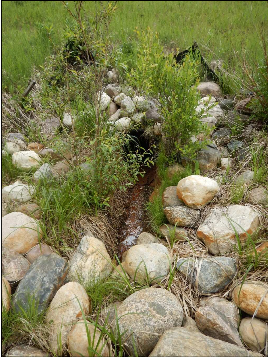
Photo 7: West culvert inlet protection well vegetated
