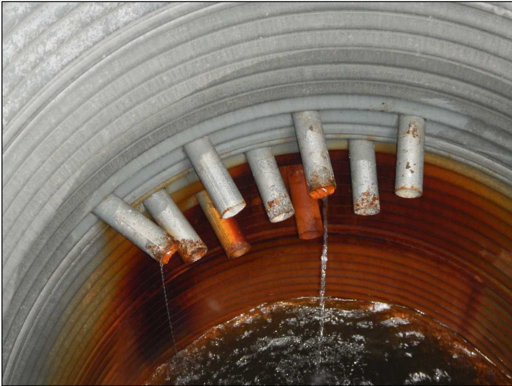
Photo 2: West drainage gallery – two of nine running
