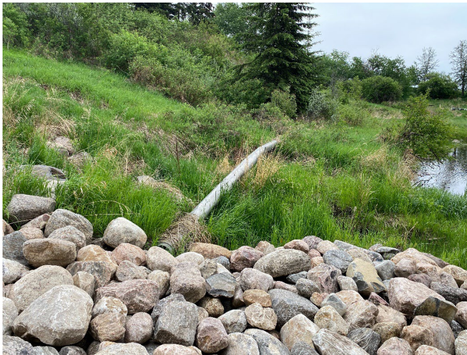
Photo 6: North ditch at C/L culvert inlet. Looking southwest.
