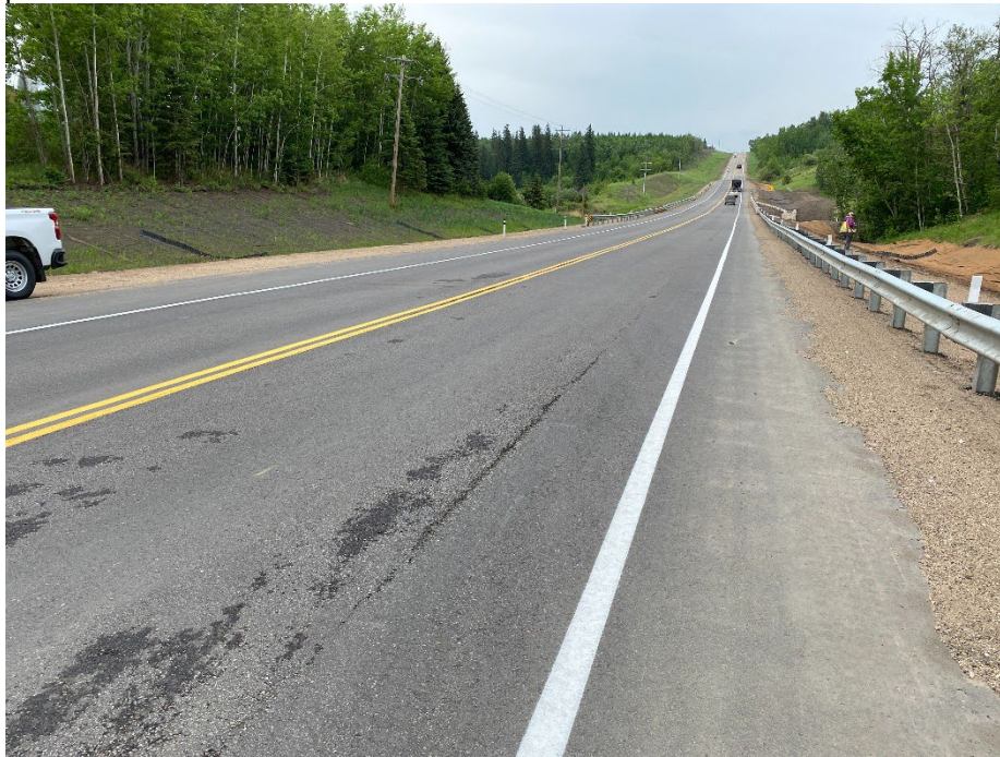
Photo 1: Highway 825, looking south.
