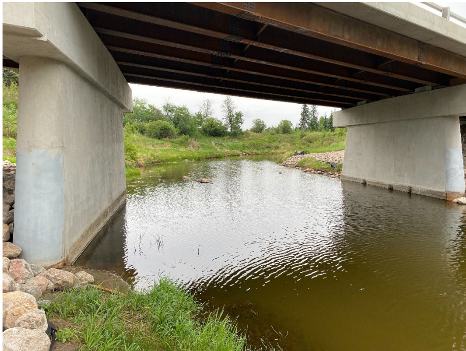
Photo 8: Condition of bridge structure after remediation activities. Looking southeast.
