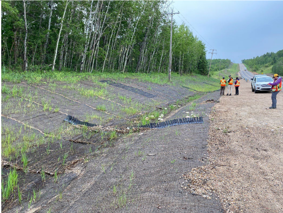
Photo 3: Erosion control blankets and georidges in east ditch, looking south.
