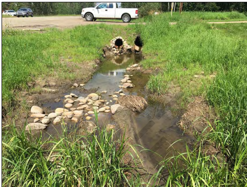
Photo 1: Standing water at culvert outlet at North Bank Potato Farm access, facing north.
