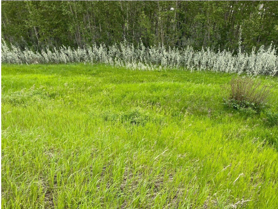
Photo 9: Bulging apparent on east sideslope at middle slump. Looking east, downslope.
