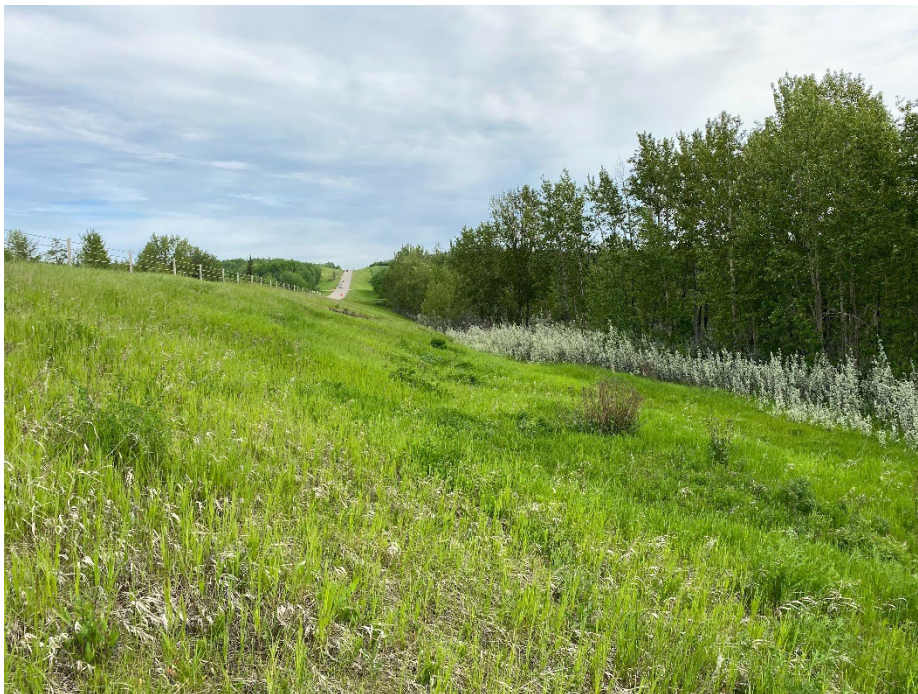
Photo 8: Middle slump on east sideslope, little change. Looking north.
