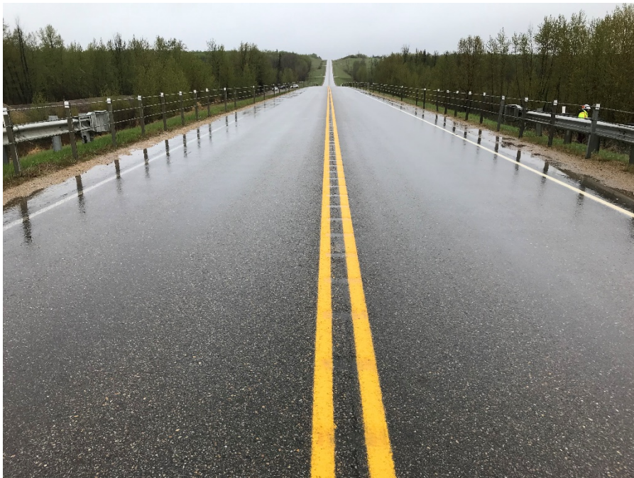
Photo 2: Pavement last milled and paved in 2016. Looking north.
