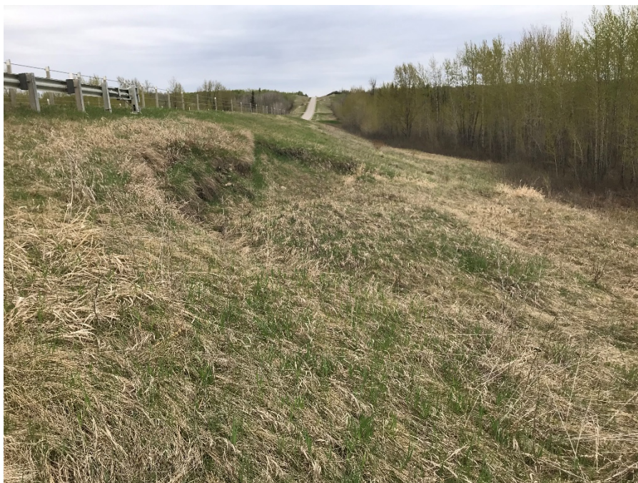
Photo 4: South slump on the east slope. Looking north.
