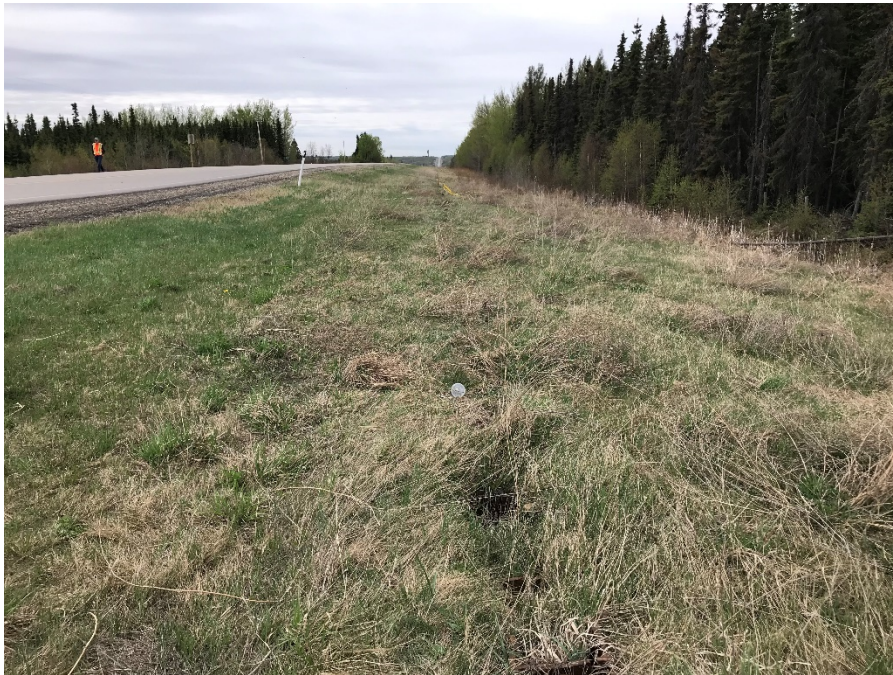
Photo 5: View of the west slope. Looking south.
