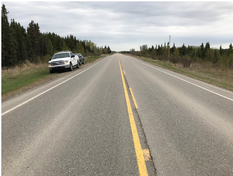
Photo 2: Highway recently paved with no observable cracks. Looking north.
