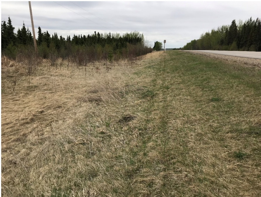
Photo 6: View of the east slope. Looking south.
