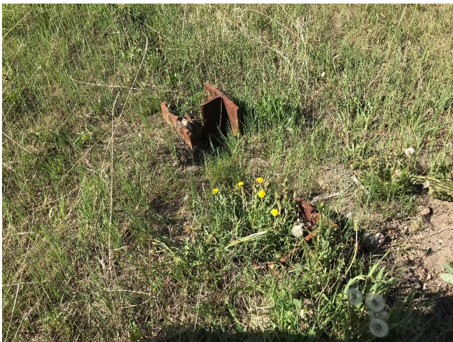
Photo 4: Exposed H-piles at the surface of the toe berm.
