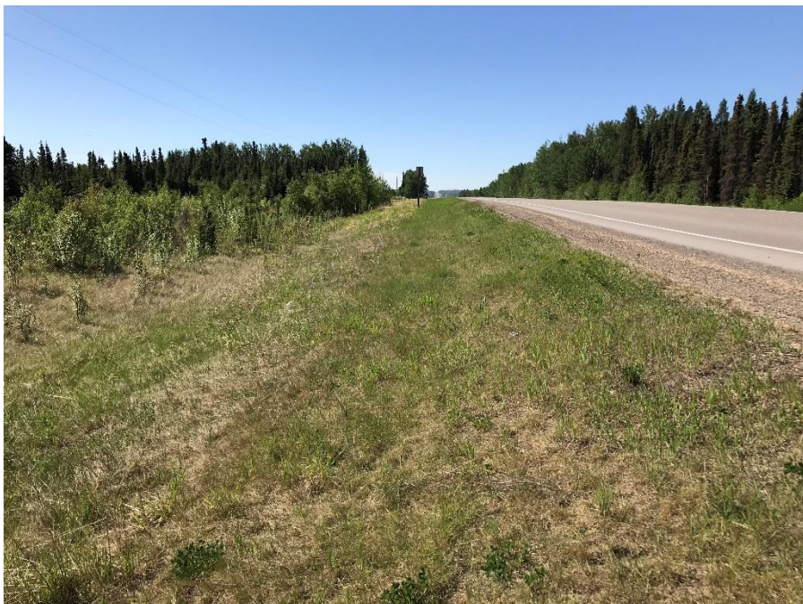
Photo 6: View of the east slope. Looking south.
