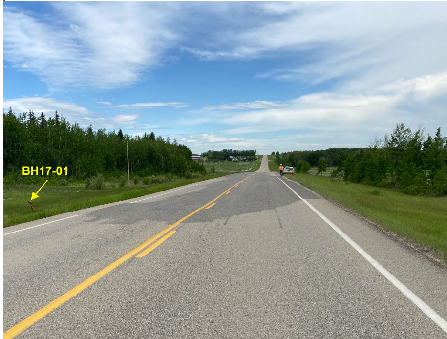
Photo 1: West extent of milled pavement. Looking east.
