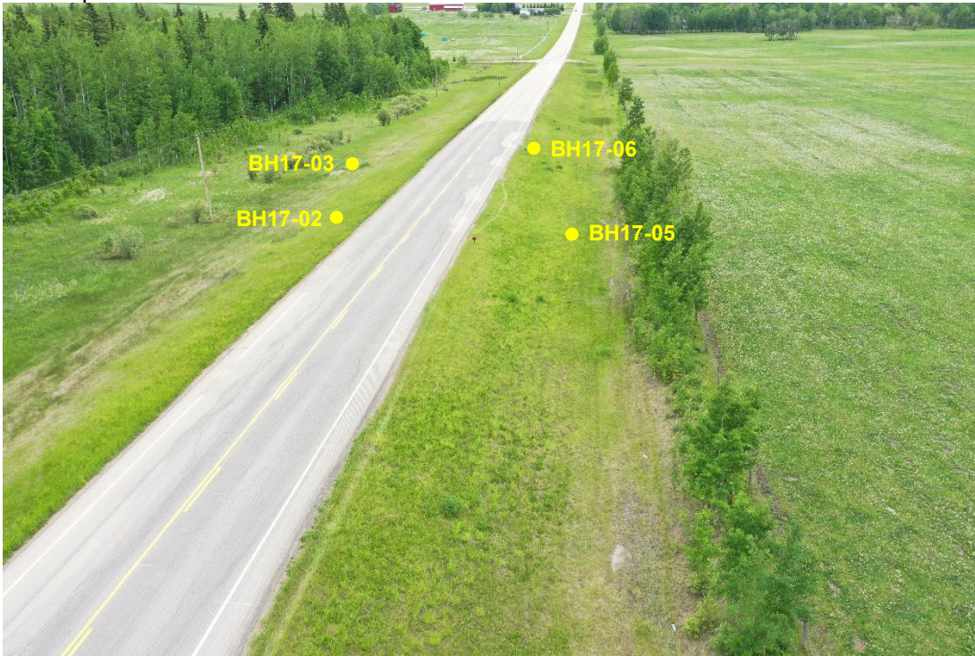
Photo 7: Site overview, taken by drone. Looking northeast.
