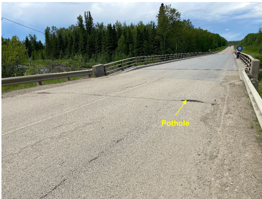
Photo 12: Pavement surface at east abutment. Looking west.
